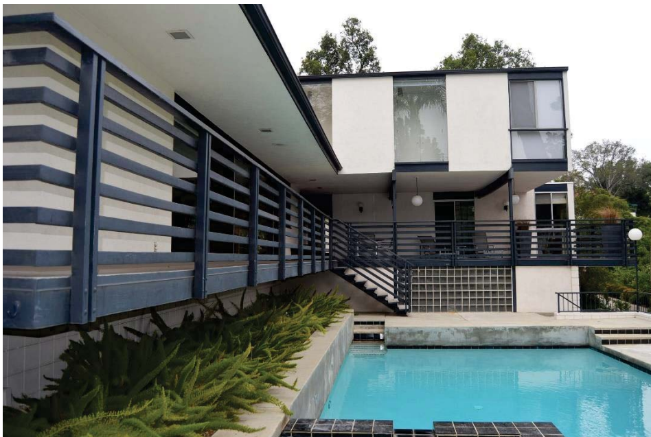
Description: Exterior, north facade View: South
