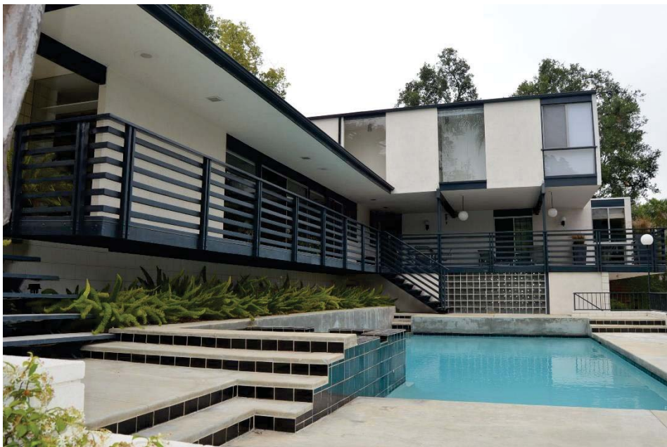
Description: Exterior, north and west facades View: South
