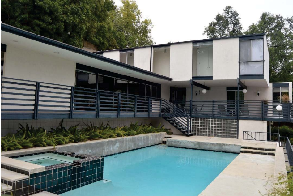
Description: Exterior, north and west facades View: Southeast
