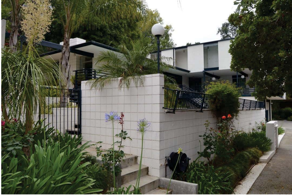
Description: Exterior View: Southeast
