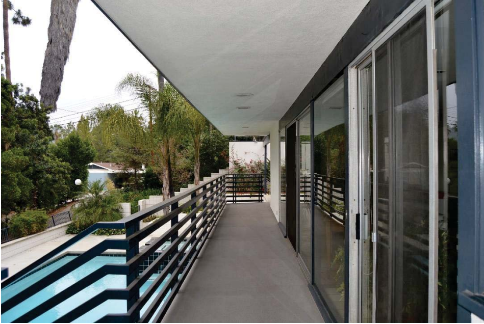
Description: Exterior, deck View: North
