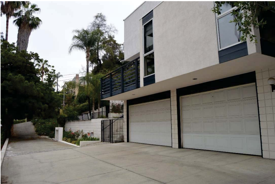
Description: Exterior, west facade View: Northeast
