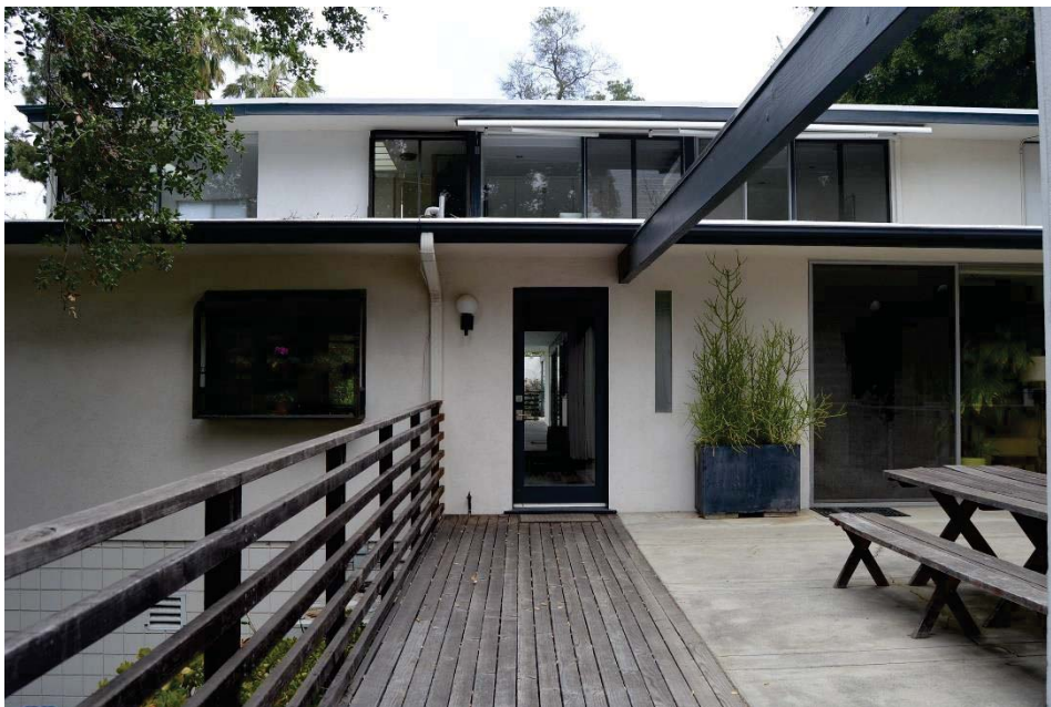
Description: Exterior, south facade View: North
