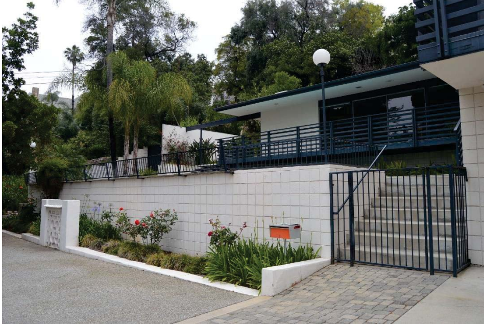
Description: Exterior, west facade View: Northeast
