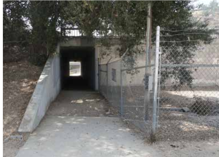
Tunnel Exterior North
