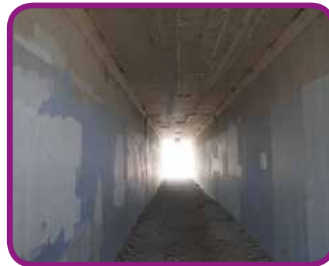
Existing tunnel Interior facing South
