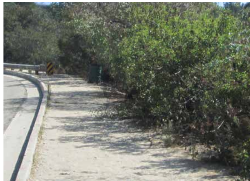
Lack of wayfinding at Lower Arroyo threshold
