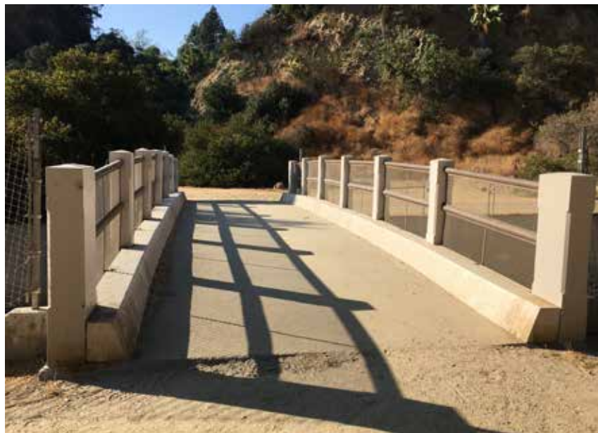
Lower Arroyo South Crossing
