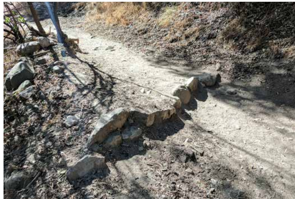
Trail Erosion & Walkability
