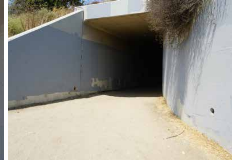
Tunnel Exterior South
