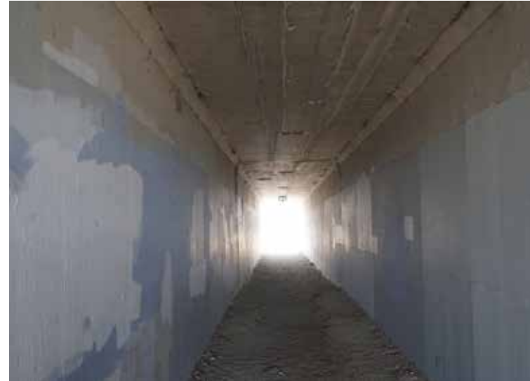
Tunnel Interior facing South
