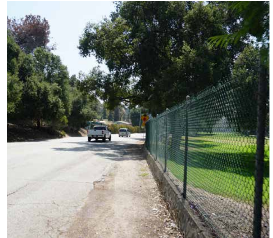
Existing condition, Rosemont Ave north of Washington Blvd
