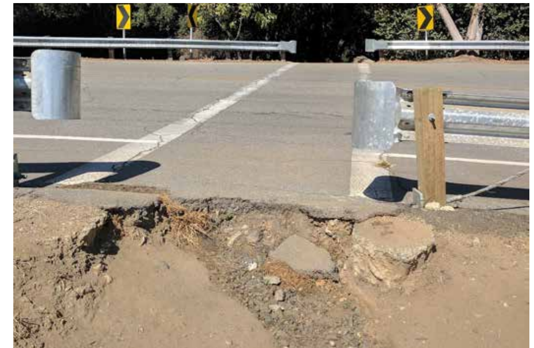
Trail Erosion & Walkability
