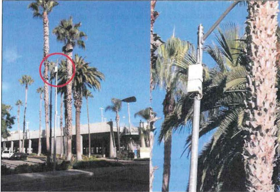
**Figure 2:** Small cell (in red circle) mounted on an existing light standard [Close up on right].
