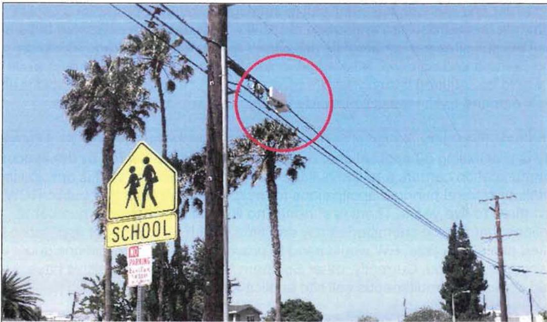
**Figure 1:** Small Cell (in red circle) mounted on a pole-to-pole strand located in the City of Torrance.
