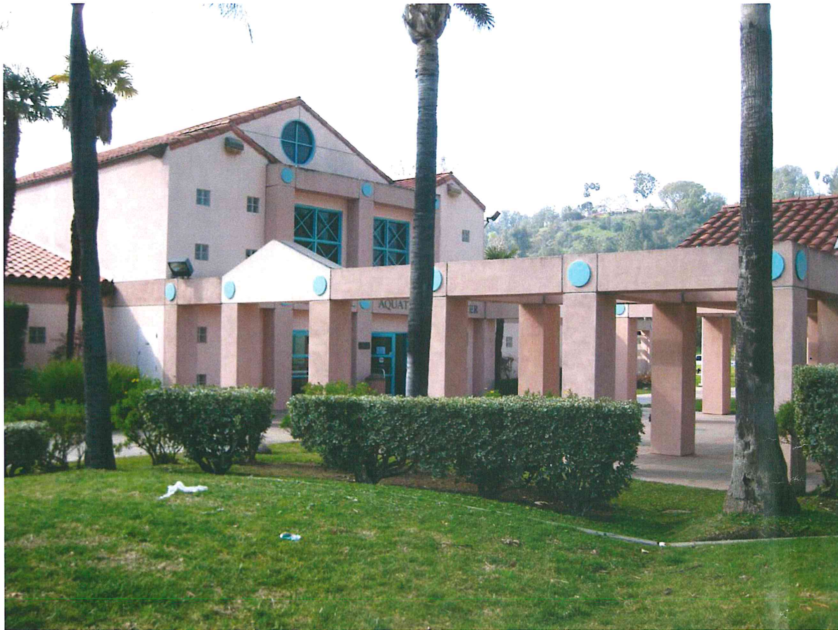
VIEW LOOKING WEST (PAST ENTRY, TOWARD PARKING LOT)
