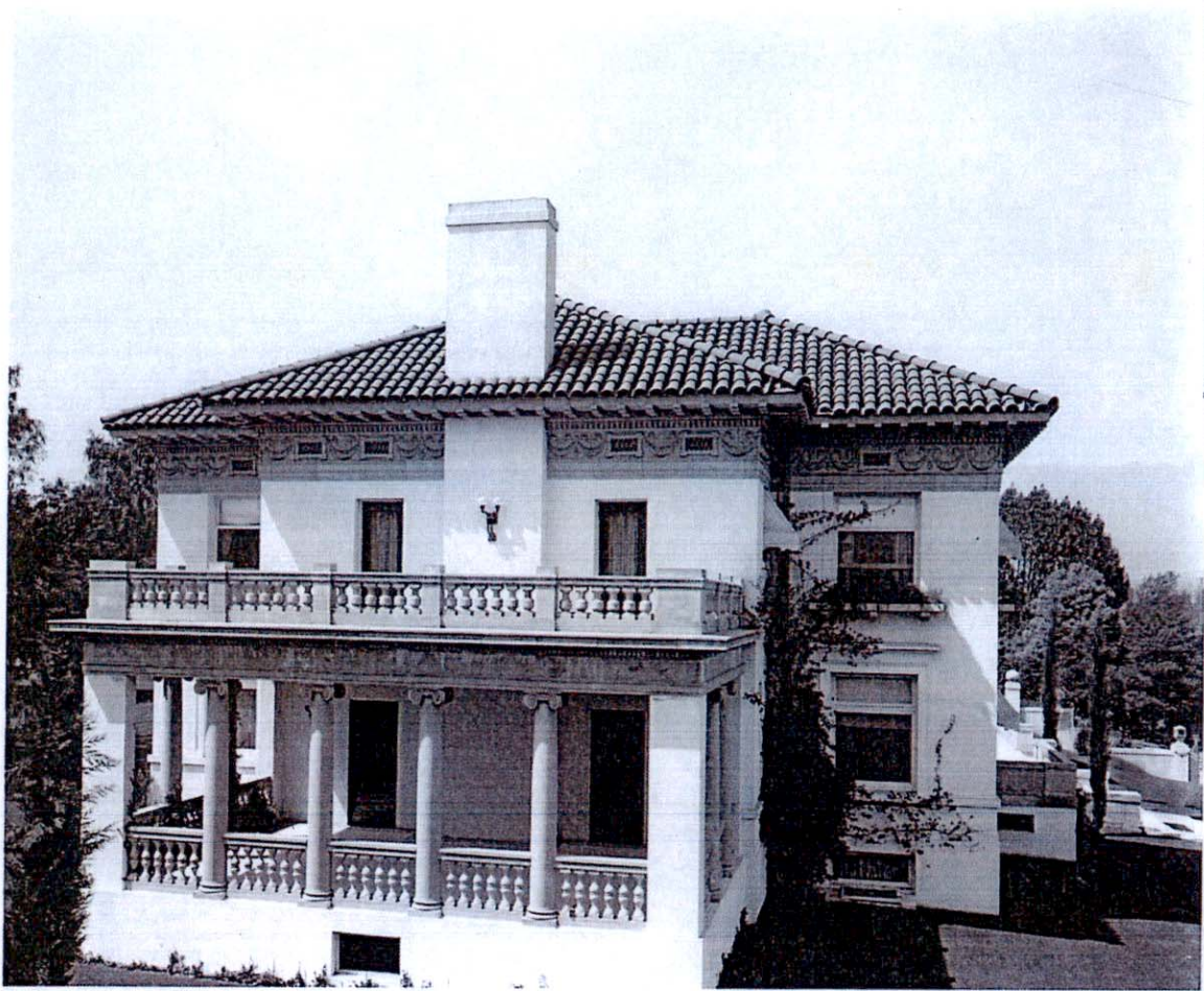
Figure 5: South façade, view facing northwest, n.d. Image courtesy of Pasadena Museum of History Archives.
