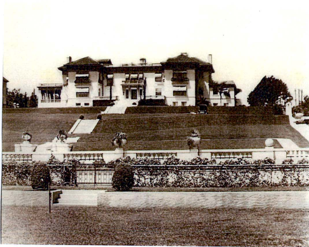
Figure 2: East façade, view facing west, n.d. Image courtesy of Pasadena Digital History Collection.
