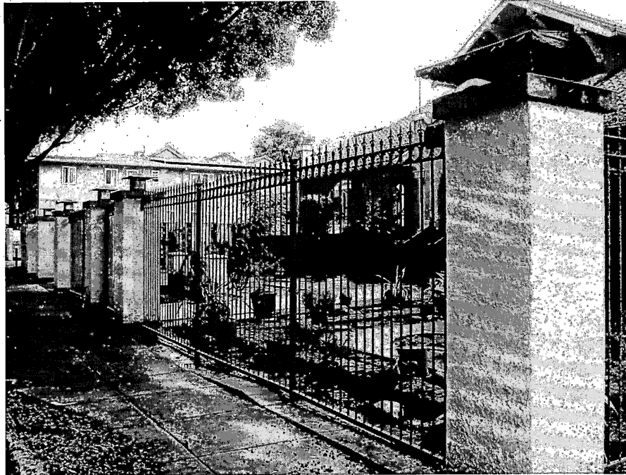
Figure 11. Looking northeast along the front yard area and sidewalk with six large piers and iron security fence.
