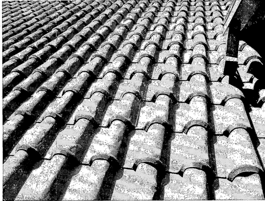
Figure 1. Looking east at the sheet metal roofing imitating a red clay tile roof, primary west elevation.
