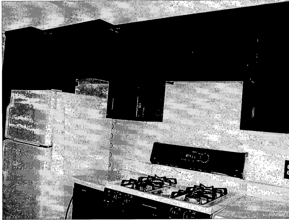
Figure 18. Looking northeast at the second-story kitchen area.
