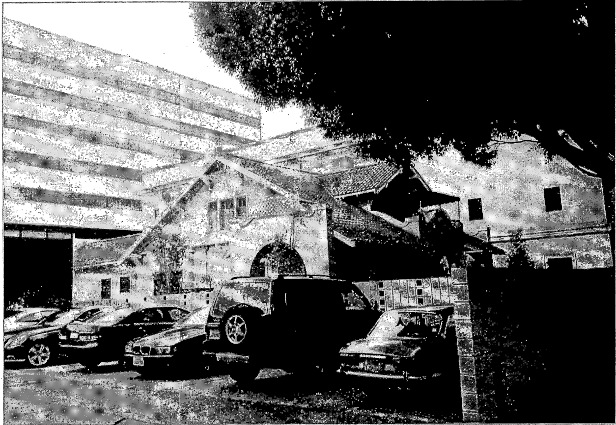
Figure 3: North Elevation. Source: GPA, November 2013.
