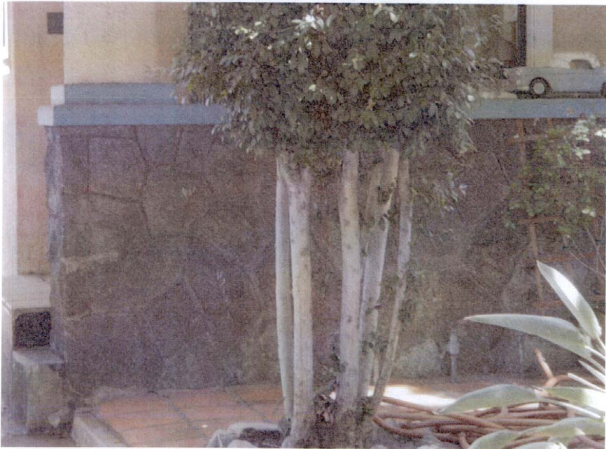
180 S. Euclid Avenue Rock Porch Wall Detail
