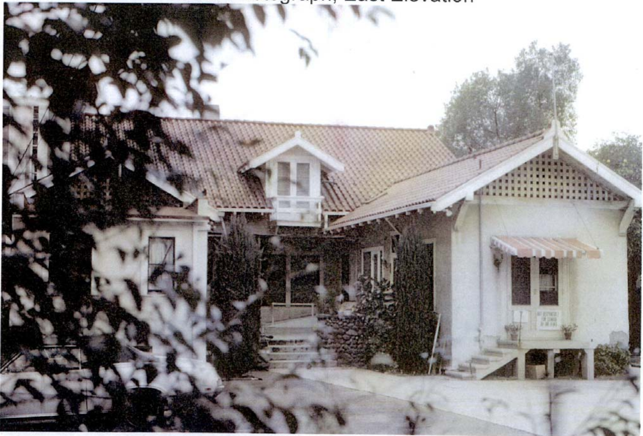
180 S. Euclid Avenue 1979 Photograph; East Elevation
