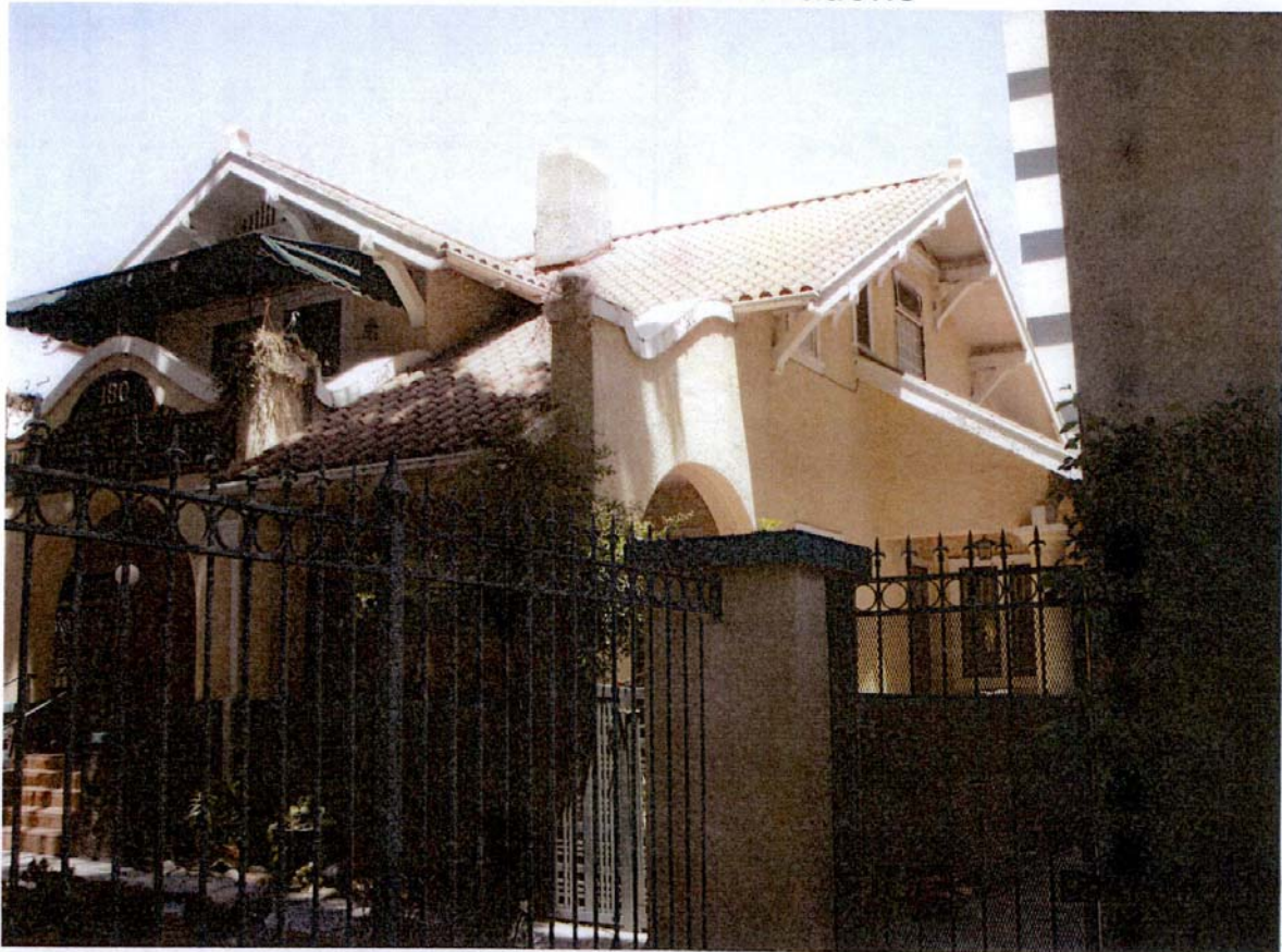
180 S. Euclid Avenue West and South Elevations
