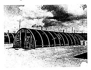
The "Portaseal® hut," frequently seen along the Alaska Highway and Canol pipeline, is mostly likely a Canadian version of the wood-framed, plywood-clad Quonset-type structure. These huts were shipped in prefabricated sections, could be erected quickly, and were heated with improvised oil drum stoves. Identifiable features include a tar paper finish nailed atop plywood sidewalls, end walls with
