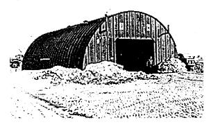
Cowin and Company, Inc. developed large, bloated, semicircular steel warehouses (slightly less than half a circle) for the Air Corps. These 36' x 60' structures were called "Steeldromes." To resist thrust on the arch caused by snow loads, Cowin used a truss system of horizontal steel tie rods and vertical steel hangers. Not many Cowin huts were shipped to Alaska after 1943 because they were inadequate for Alaskan snow loads. A number of them collapsed in their first winter of use.
