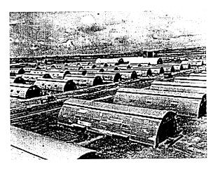
The last major redesign of the Quonset hut came in about 1943 when the factory at Quonset Point was phased out and the contract to produce Quonset huts transferred to the Stran-Steel Division of the Great Lakes Steel Corporation. The new hut had an expanded footprint of 20' x 48' and reverted back to the full arch rib.
