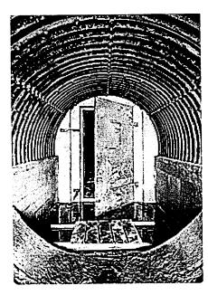
During World War II, the Armco International Corporation of Middletown, Ohio, produced arched corrugated ingot iron bunkers, ammunition magazines, and personnel shelters. The heavy steel buildings were modeled on earth-retaining structures such as culverts and storm sewers. The heavy iron (8- to 14-gauge) did not require supporting ribs but was curved and corrugated much like a Quonset hut." Armcos" were strong enough to be completely buried in up to six feet of dirt.
