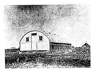
Since the arch of the Quonset hut extended to the floor, beds, sinks, and washing machines had to be moved inward until they abutted the curve at the top edge of the unit. Valuable floor space was being wasted. Reclaiming this space would necessitate changing the overall form of the building.
