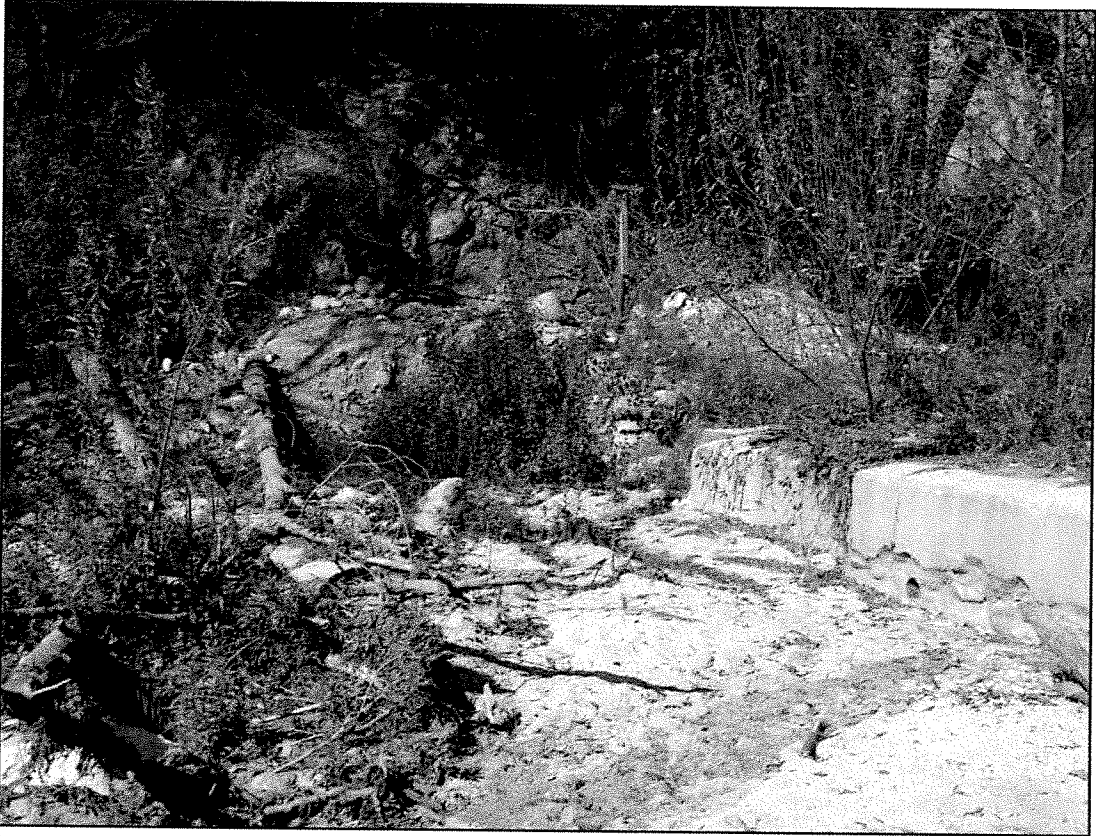
Figure 8. Wildlife can easily pass over and around existing diversion structure in Area 2.
