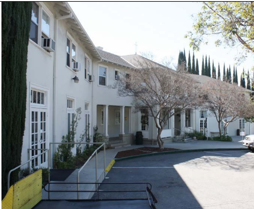
Current appearance of Administration Building. (ARG, 2/2015)
