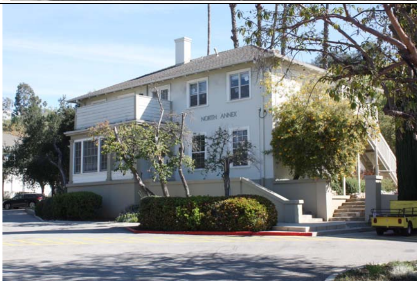
Current appearance of North Annex, view northeast (ARG, 2/2015)
