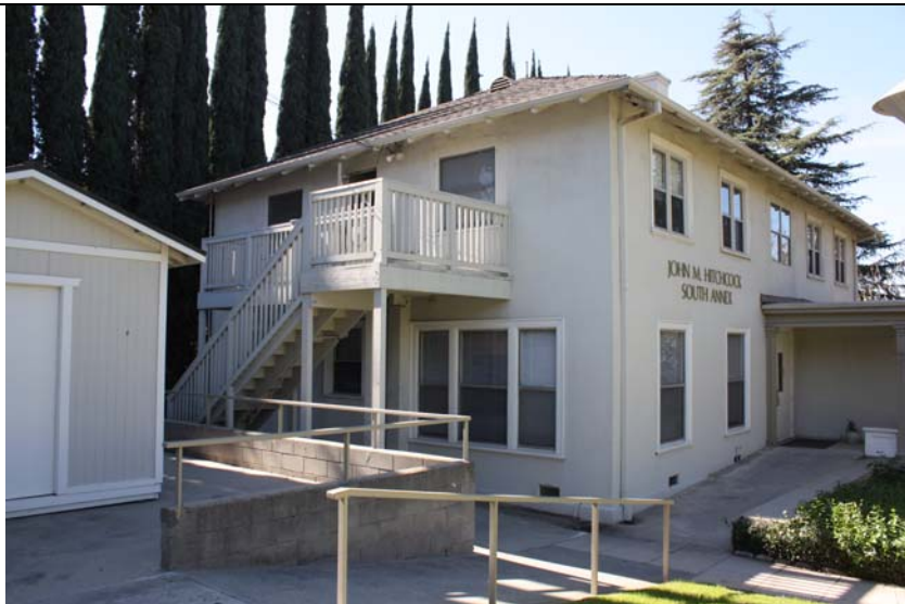
Current appearance of South Annex, view west of side façade (ARG, 2/2015)
