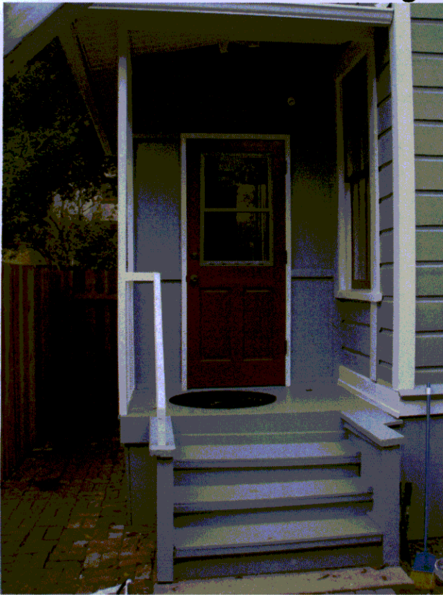
Easterly Service Porch
