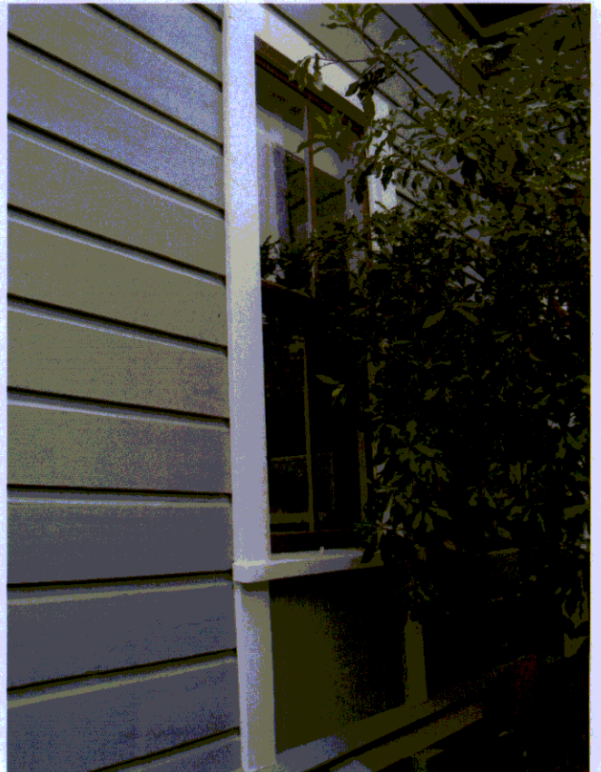
Window at Rear Porch Enclosure
