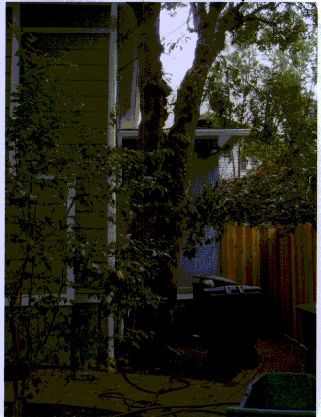
Enclosed Rear Porch - West Elevation
