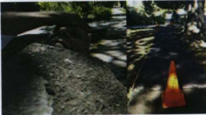
L.A.'s Broken Sidewalks
