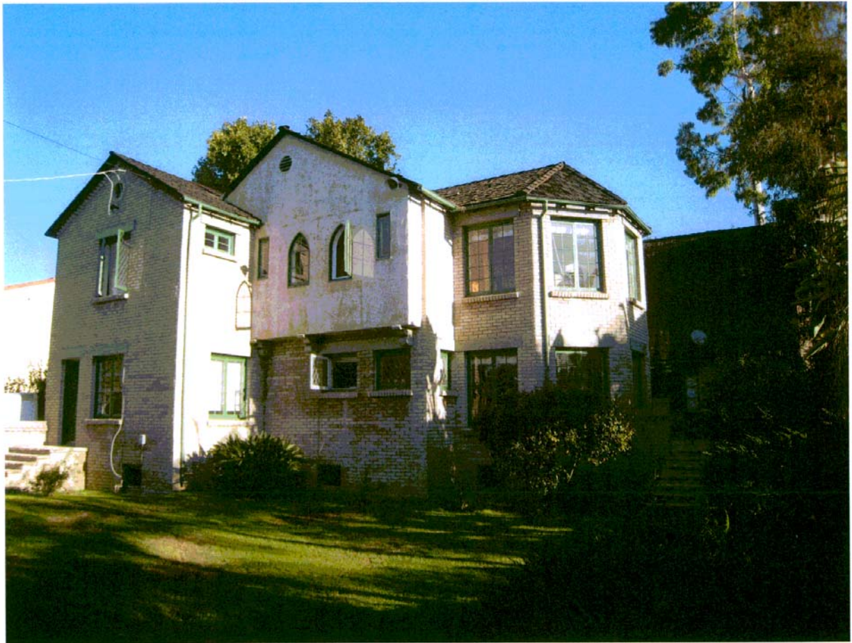
Central Portion of Rear Elevation
