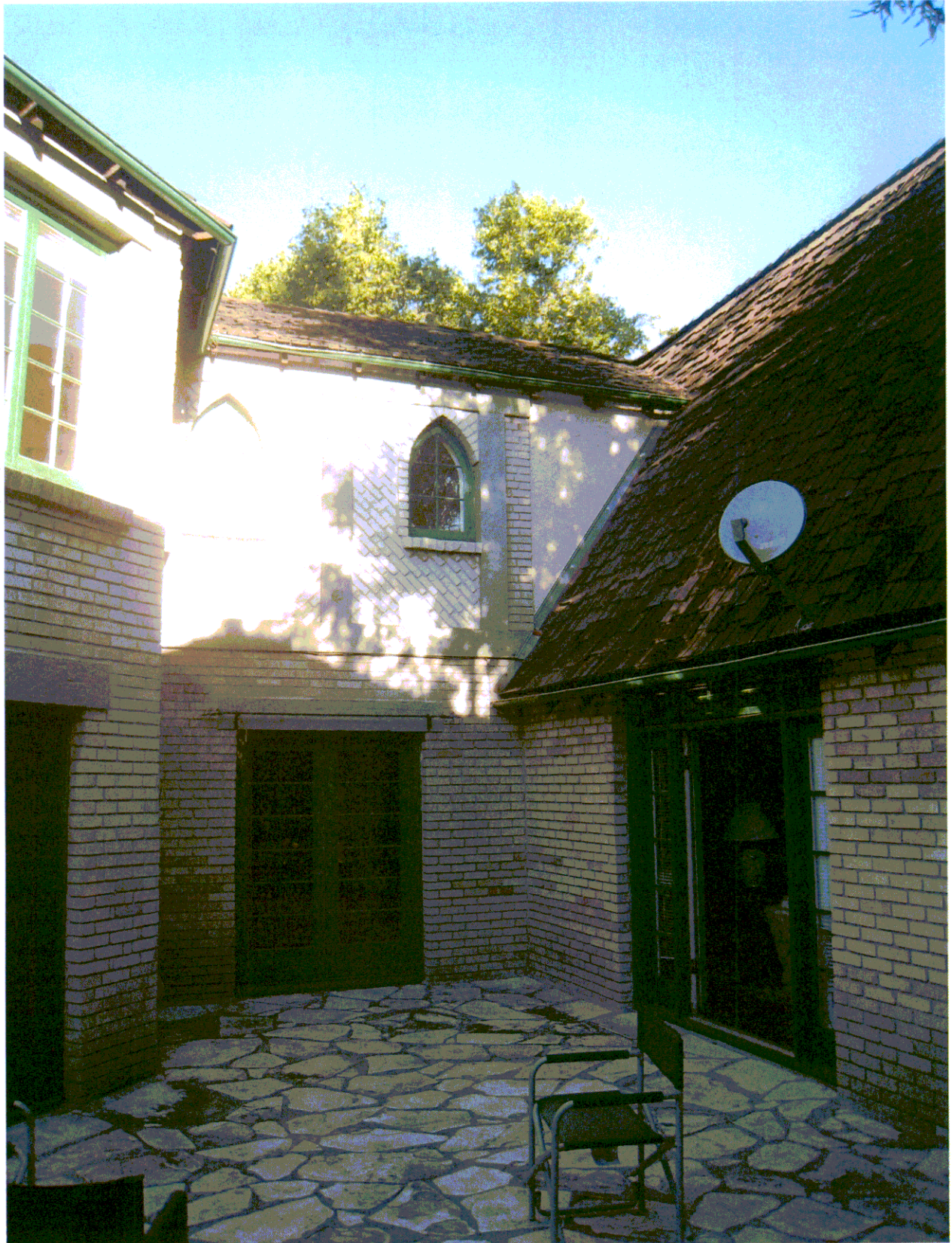
Portion of East Elevation
