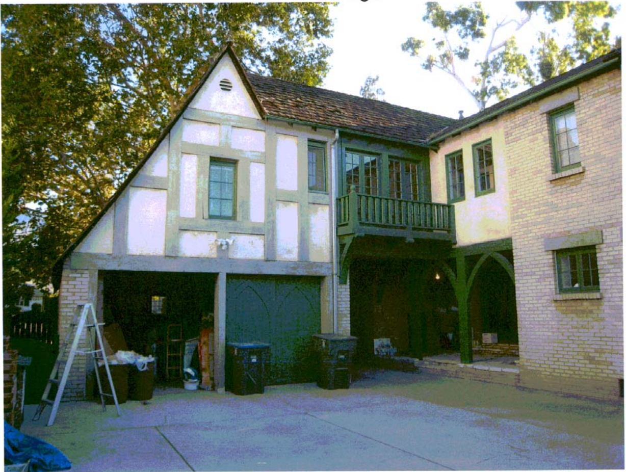
Rear of Garage
