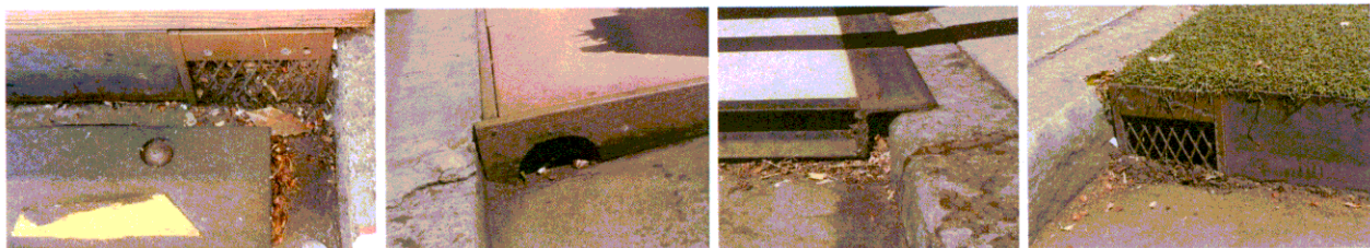
Drainage channel outlets may pose maintenance issues if not designed and maintained properly
