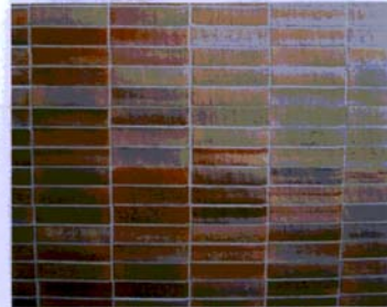
WALL TILE | The materialistic quality of this element helps support the character defining features of the architecture. Used as a main exterior wall 'in fill' finish in limited applications to define mass at the corners of the building. Note the variance in tone, size and pattern of the tiles.
