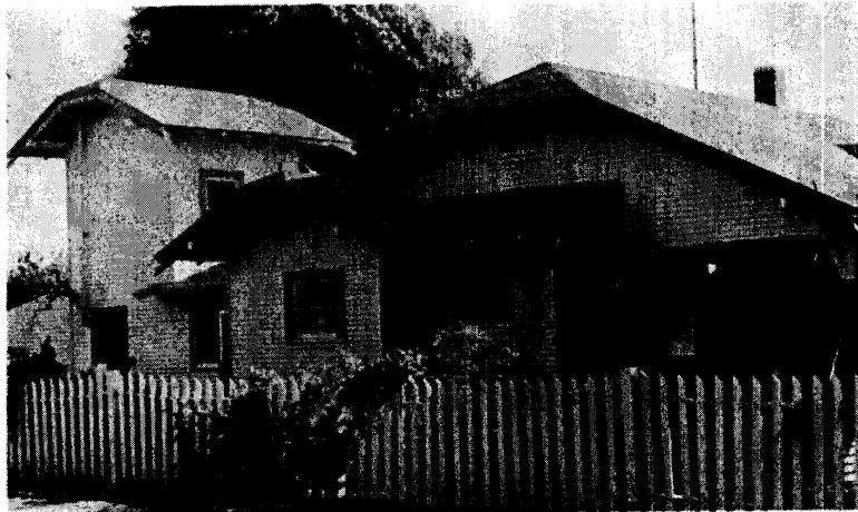
FIGURE 10. The hipped roofs of the house and tankhouse exhibit an architectural blending on this example near Ripon, San Joaquin County. The tankhouse in this case is attached to the house and is accessible from inside the house. Attaching the tankhouse to the house became common after 1910.
