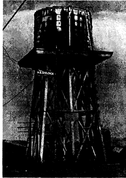
FIGURE 1. Skeletal tower and elevated water tank on a farm near Hollister, San Benito County, California. Most California farmers considered an exposed tower such as this unsightly and preferred to enclose it to form the more useful tankhouse.
