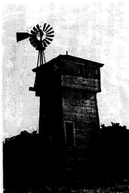
FIGURE 4. Straight box tankhouse near Turlock, Stanislaus County, typifying the most common and widespread of all tankhouse types in California, and representing the type most prominent in the Sacramento and San Joaquin Valleys.
