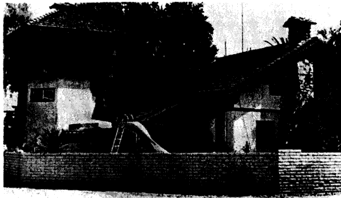
FIGURE 14. This tankhouse attached to a house near Modesto, Stanislaus County, has been stylized to blend architecturally with the house. Though it is octagonal in shape, it is basically a tapered-tower overhang type.
