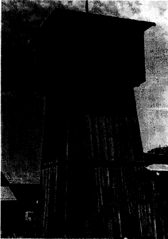
FIGURE 12. Board-and-batten construction, Bear Valley, Mariposa County, built about 1935 by a CCC crew. The ground floor was used as a shower room for miners.
