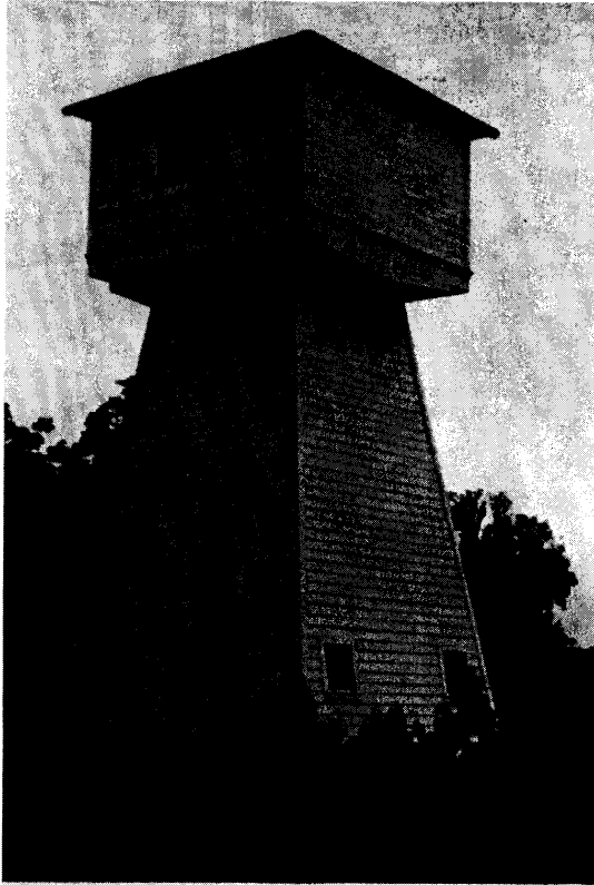
FIGURE 8. Tapered-tower overhang on the Rossi Vineyards near St. Helena, Napa County. The tower supports on this example are tapered more than is typical. It was built before 1900 and contains a 5,000-gallon redwood water tank.
