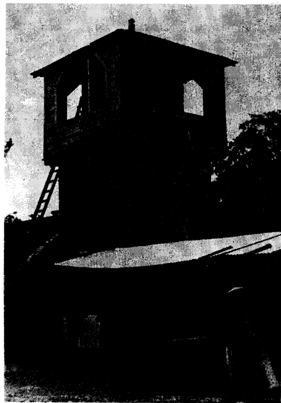
FIGURE 9. Common in both the rural San Francisco Bay and Monterey Bay areas are tankhouses having partially-walled tankrooms. This example is near Gilroy, Santa Clara County.
