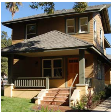
Heritage Partners Restoration
