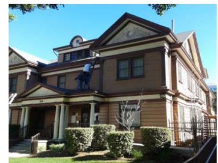
Euclid Villa Rehabilitation
