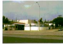
8. COMMERCIAL BUILDING (241 N. ALLEN) NORTH OF PROPOSED SITE
