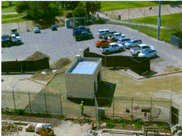
Broadcast Building Overhead, March 28, 2013 Last Month
