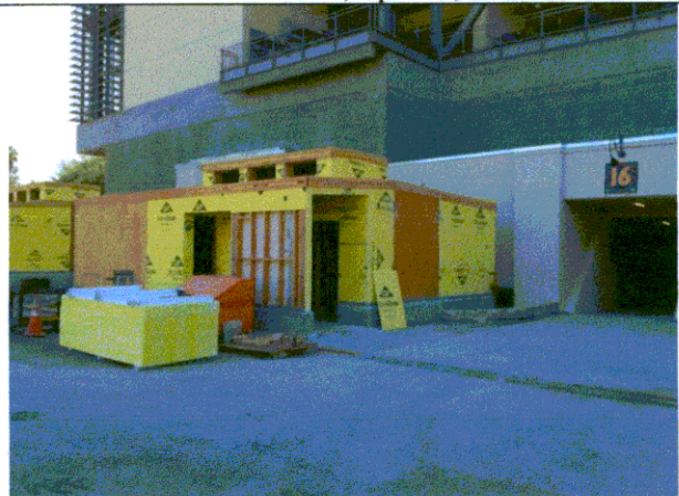
Restroom AE-12, April 26, 2013
