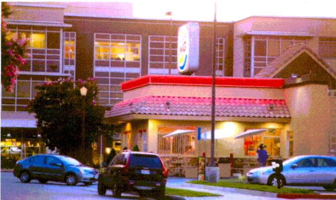
Fair Oaks —Burger King facing Fair Oaks. North of this property is the former Monty's (now a parking lot) and Grandview Palace, which will likely be a medical office building at some point.
