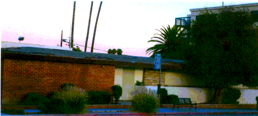
Raymond Ave—This dilapidated property is immediately adjacent to the Fillmore station.
