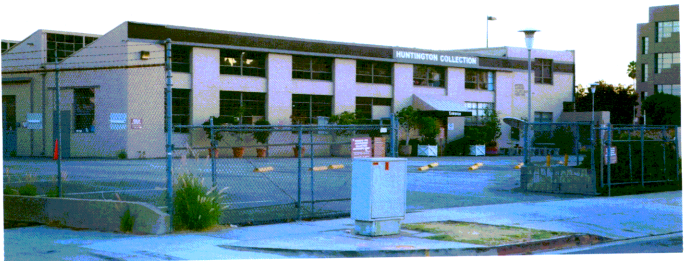
Fillmore Ave —Facing S Fair Oaks Ave.
