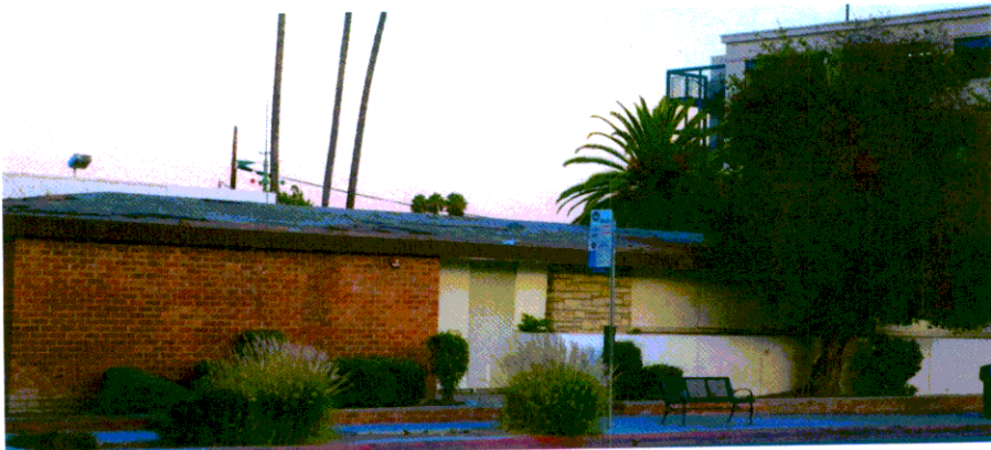
Raymond Ave —This dilapidated property is immediately adjacent to the Fillmore station.
