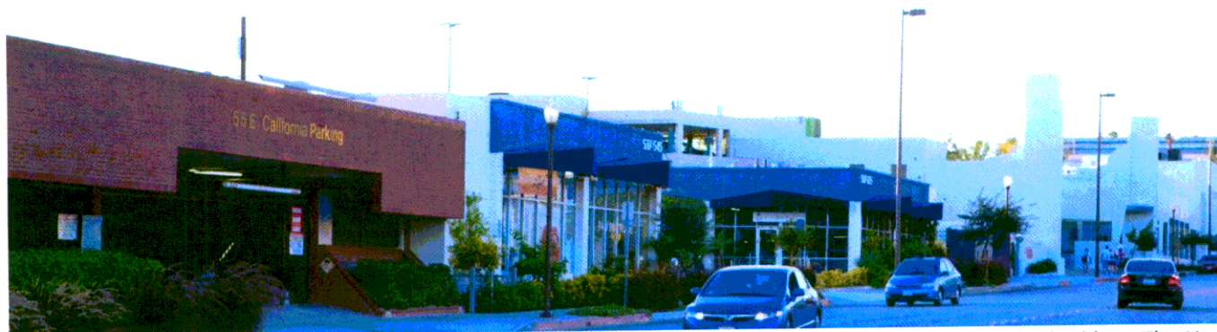
Raymond Ave & California —Looking north. At the right of the photo is the Disney Story/Royal Laundry building. The U-Haul lot and storage facility is across the street.
