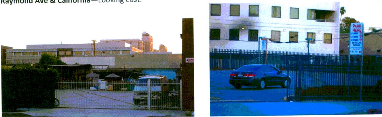
Raymond Ave —South of California. Despite being adjacent to the Fillmore Gold Line station, these properties are industrial. The “Bio-Tech” vision of the last several decades never emerged.
