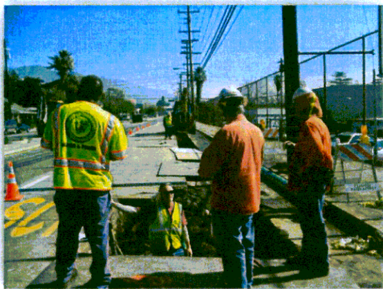
Example of 24-Inch Pipeline Trenching
