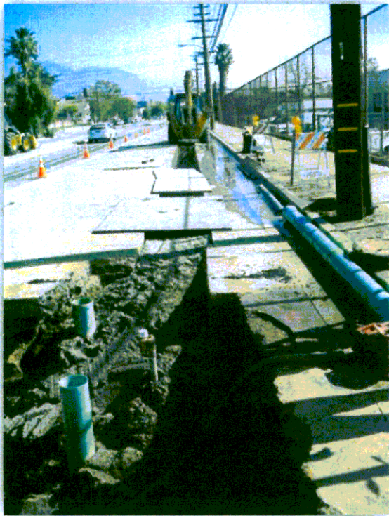
Example of 24-Inch Pipeline Trenching
