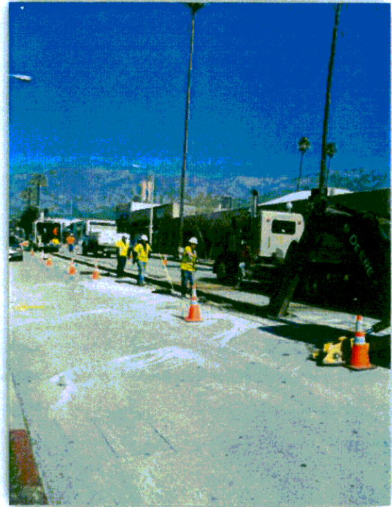
Example of 12-Inch Pipeline Installation
