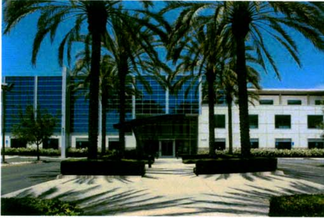
GDC Building, Pasadena
