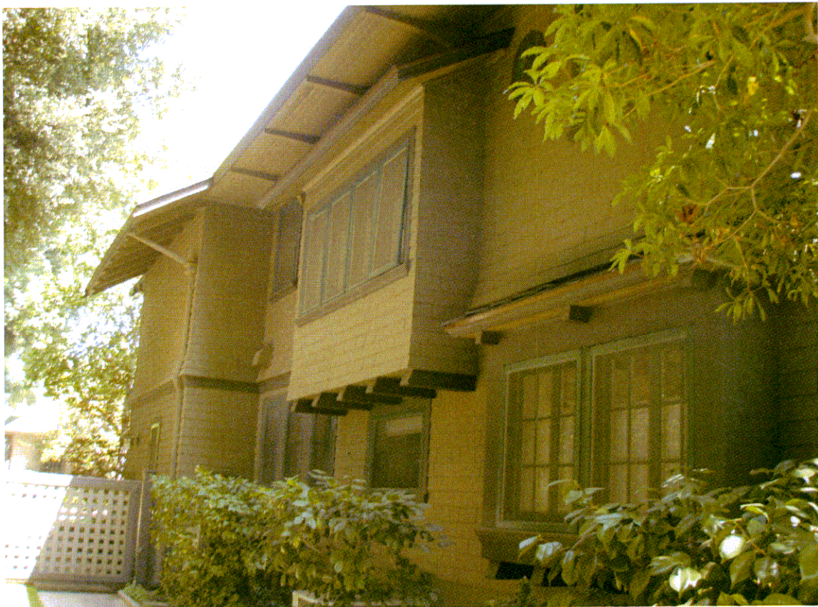
CA_Los Angeles County_George B Post House_0004
