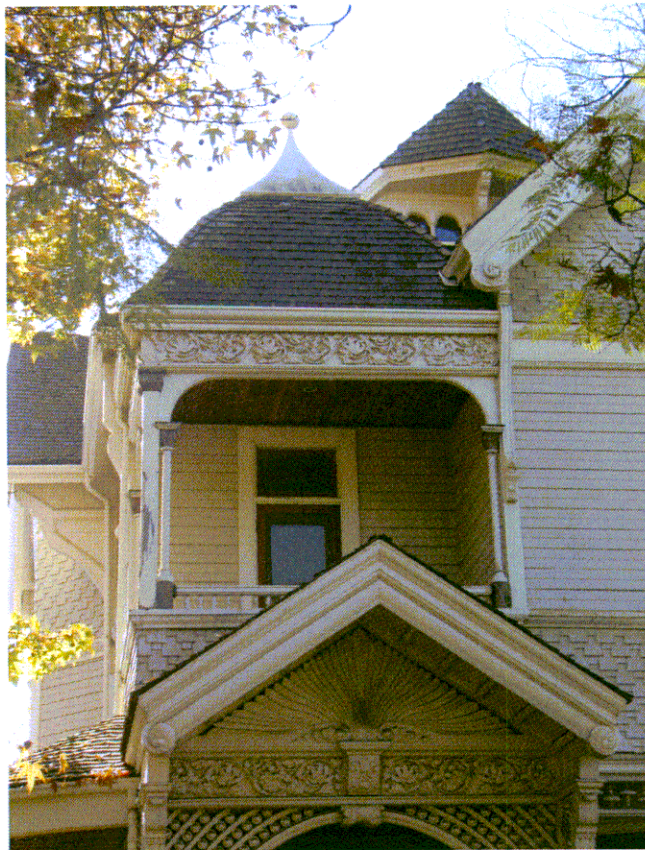
CA_Los Angeles County_James F Cosby House_0004
