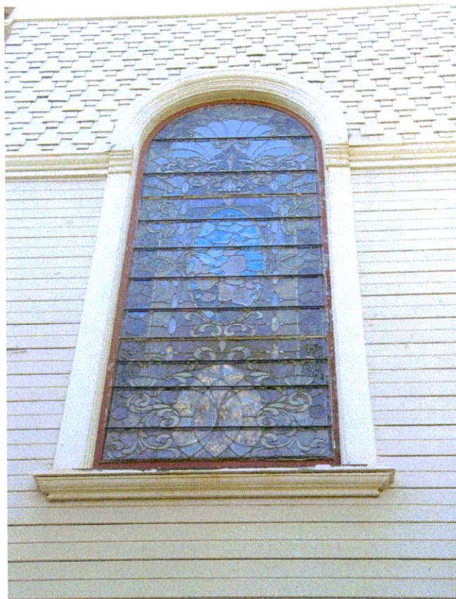
CA_Los Angeles County_James F Cosby House_0009
