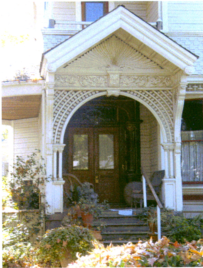
CA_Los Angeles County_James F Cosby House_0003
