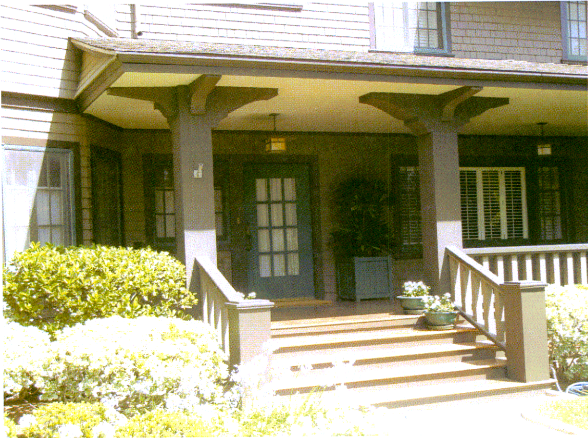
CA_Los Angeles County_George B Post House_0003
