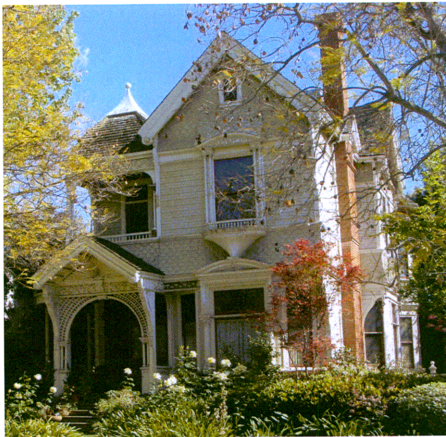
CA_Los Angeles County_James F Cosby House_0001
