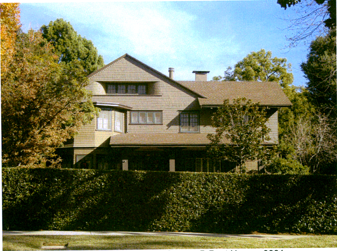
CA_Los Angeles County_George B Post House_0001
