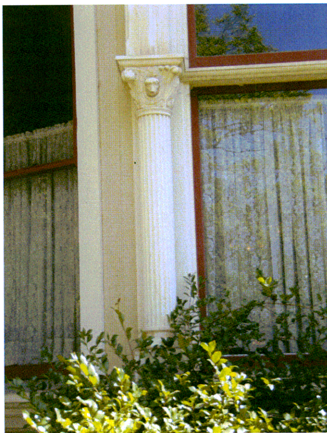
CA_Los Angeles County_James F Cosby House_0006
