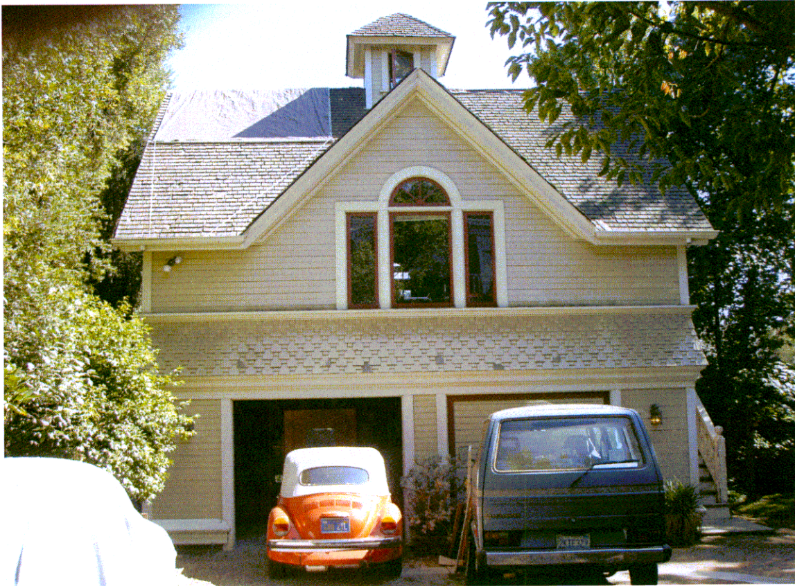
CA_Los Angeles County_James F Cosby House_0011
