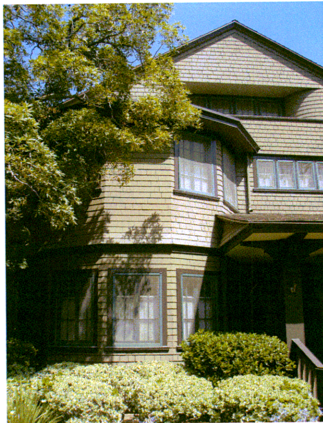
CA_Los Angeles County_George B Post House_0002
