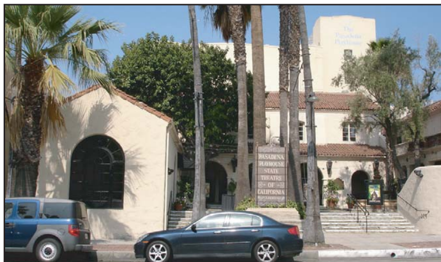
Photo 7 - View west from the project site, across El Molino Avenue, of the Pasadena Playhouse and Playhouse courtyard.
