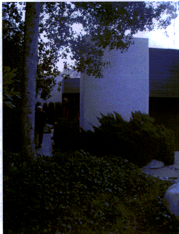
Westerly portion of garage; main entry behind
