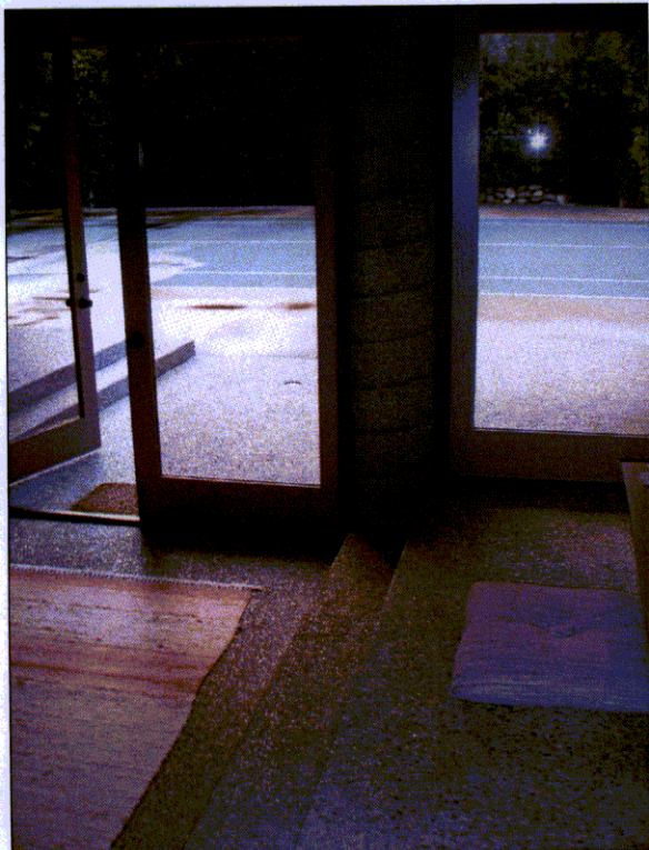
Detail of pavilion flooring, terrace & pier material
