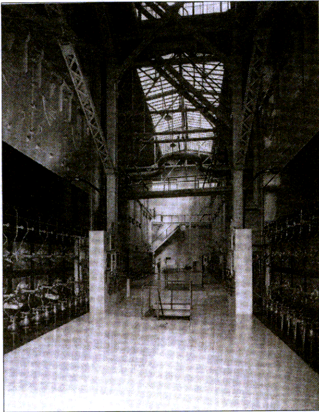
Boiler Room hallway (east end – now empty)
