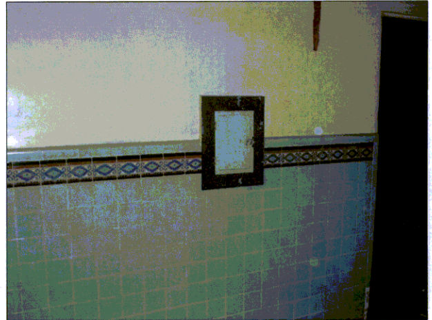
Turbine Hall tile detail
