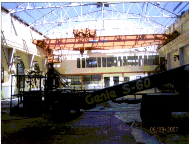
Easterly portion of Turbine hall
