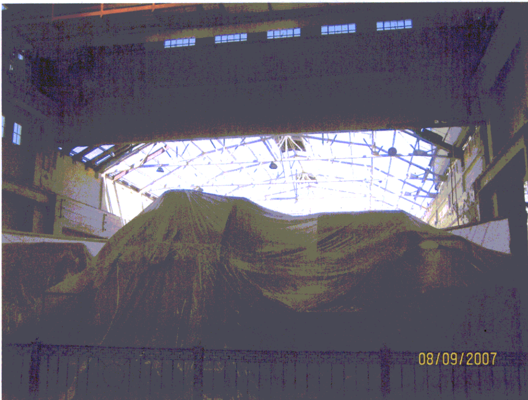
Turbine Unit 8 (current)
