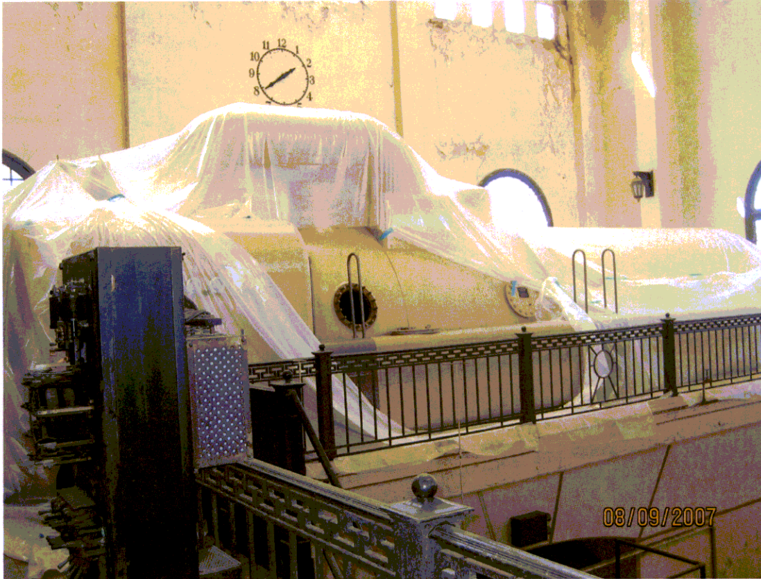
Turbine Unit 9 (current), clock and railing
