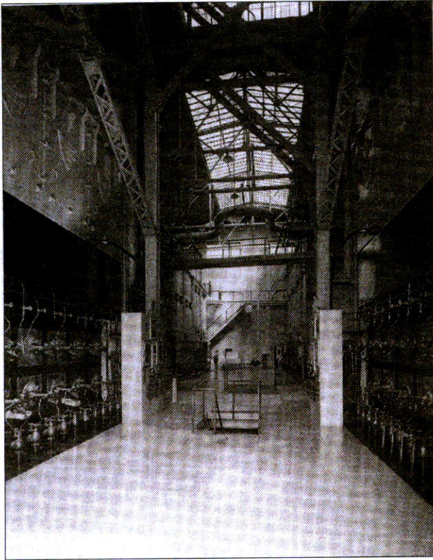
Boiler Room hallway (east end – now empty)
