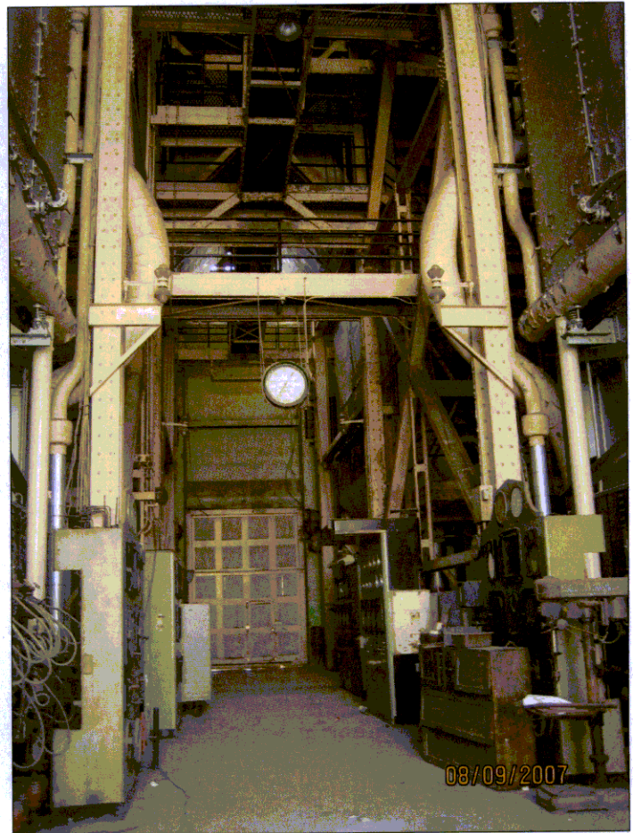
Boiler Room hallway (west end - current)
