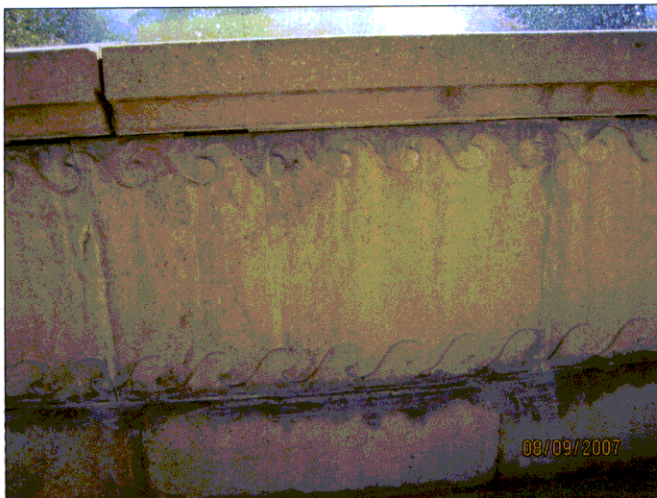
Fountain perimeter wall detail
