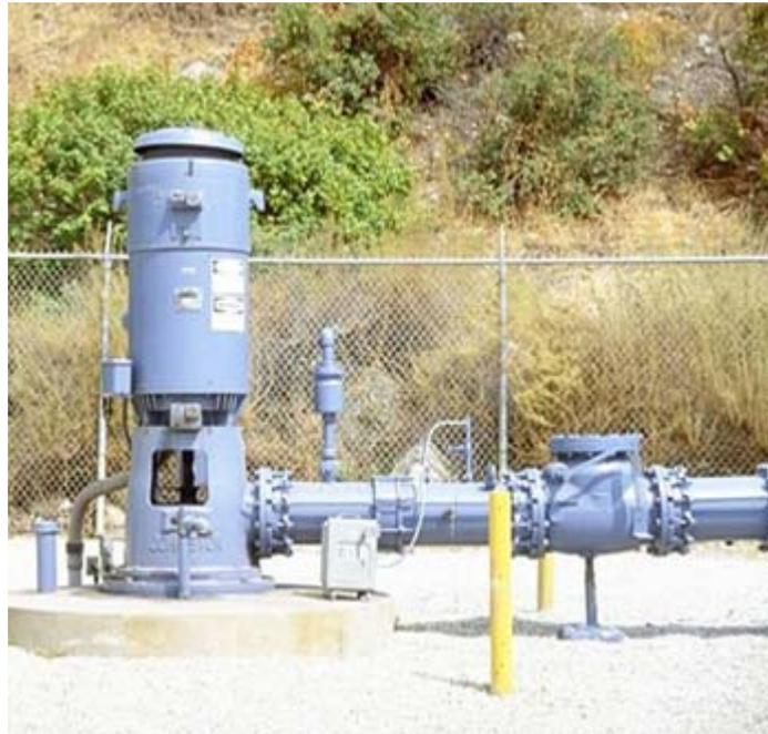
**DESCRIPTION:** This project provides for the upgrading or replacing of older and less efficient well and booster pumps, and obsolete and outdated switchgears.
