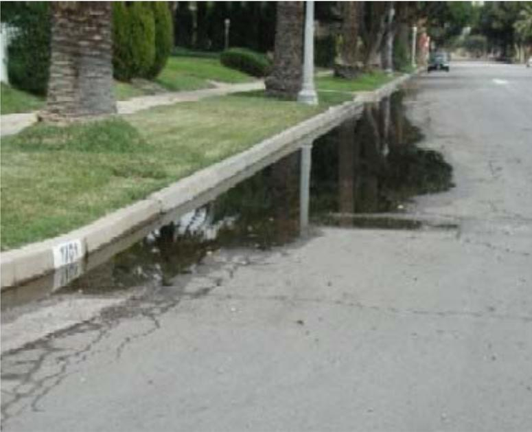
**DESCRIPTION:** This project provides for drainage improvements on streets with flat grades throughout the City. The work involves the reconstruction of curb, gutter, and pavement as necessary to correct drainage problems.
