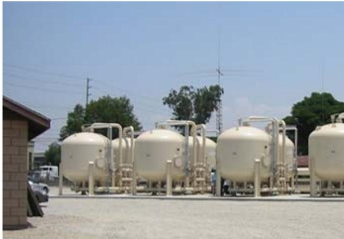
**DESCRIPTION:** This project provides for the design and construction of a perchlorate treatment system for the Monk Hill wells. The plant will treat Arroyo, Well 52, Windsor and Ventura wells. Perchlorate was first detected June 1997, and by January 2002 all four wells were shut down when the State lowered its action level for perchlorate.
