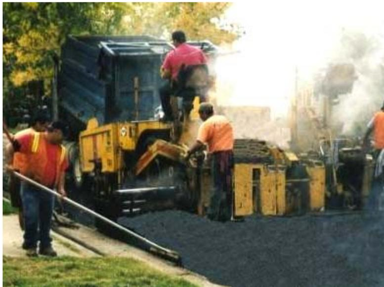
**DESCRIPTION:** This project provides for the systematic resurfacing (asphalt overlay) and slurry sealing of all asphalt streets throughout the City at prescribed intervals. These intervals vary depending on the age of the street and traffic volume. This project also includes funds for a separate project to repair damaged concrete adjacent to the street to provide proper drainage and better ride quality.
