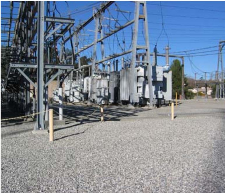
**DESCRIPTION:** This project provides for the construction of oil containment systems at all substations that will prevent any mineral oil spills from the transformers and electrical equipment from affecting the environment.
