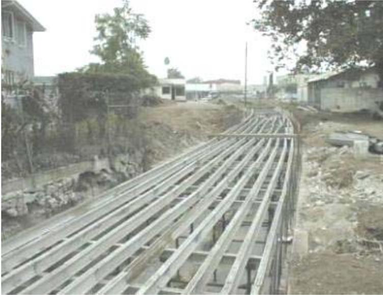
**DESCRIPTION:** This project provides for the improvement of the East Side Storm Drain between Colorado Boulevard and the North City Limits. Phase I, which was completed in FY 1993, included structural repairs to the soffit of the drain. Phase II involves the covering of various reaches of the channel listed below. (Note: There was no Phase II-I).
