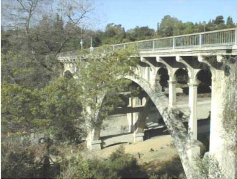
**DESCRIPTION:** The project provides for the rehabilitation of the La Loma Road Bridge that spans the Arroyo Seco at La Loma Avenue. The rehabilitation of the bridge includes seismic retrofitting, repair of deteriorated and damaged surfaces, and replication of the historical lighting and bridge rail features.
