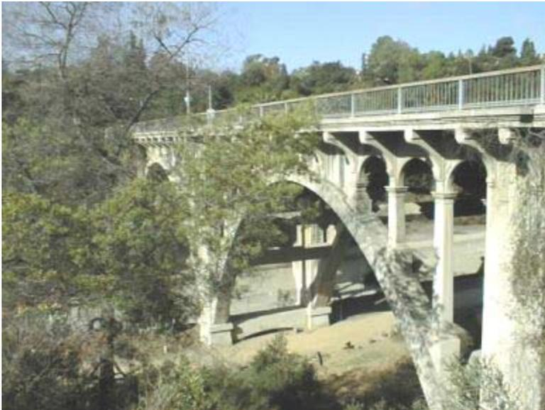
**DESCRIPTION:** This project provides for the systematic maintenance of the City's bridge structures. Bridge maintenance includes: Repair of concrete spalls and cracks; replacement of deteriorated steel reinforcement; replacement of deteriorated or missing expansion joint material; installation of grouted riprap slope protection; repair and painting of metal handrails; replacement of deteriorated asphalt overlays; and other miscellaneous work.
