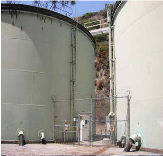
**DESCRIPTION:** This project will provide for major repairs and upgrades to the City's 15 existing water tanks and reservoirs. Most of the tanks and reservoirs are over 60 years old. Examples of the repairs and upgrades may include replacement of reservoir roofing, lining the reservoir floor with hypaton liners, and changing old outlet and inlet valves.
