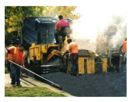
**DESCRIPTION:** This project provides for the systematic resurfacing (asphalt overlay) and slurry sealing of all asphalt streets throughout the City at prescribed intervals. These intervals vary depending on the age of the street and traffic volume. This project also includes funds for a separate project to repair damaged concrete adjacent to the street to provide proper drainage and better ride quality.
