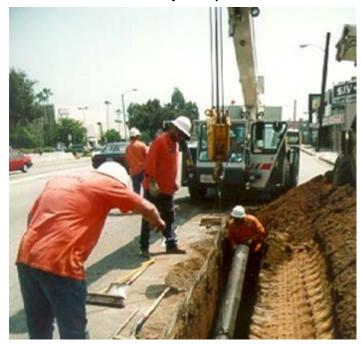
**DESCRIPTION:** This project provides for the upgrade of the water distribution system, as necessary, to sustain current fire protection requirements. Typical projects include new mains and new fire hydrants.
