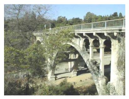
**DESCRIPTION**: This project provides for the systematic maintenance of the City's bridge structures. Bridge maintenance includes: Repair of concrete spalls and cracks; replacement of deteriorated steel reinforcement; replacement of deteriorated or missing expansion joint material; installation of grouted riprap slope protection; repair and painting of metal handrails; replacement of deteriorated asphalt overlays; and other miscellaneous work.
