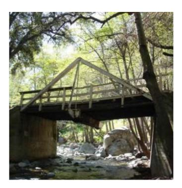
**DESCRIPTION:** This project provides for the repair of the Arroyo Seco Bridge B-4 located approximately 0.75 mile north of JPL in the Arroyo Seco. The bridge is over 60 years old and is owned and maintained by Pasadena Water and Power. It is mainly used by hikers, bikers, Fish and Game, and the U.S. Fire Service (USFS). The bridge was damaged in the 2005 winter rainstorms.
