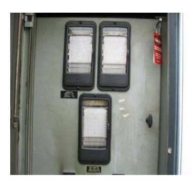
**DESCRIPTION:** This project provides for the procurement and installation of electronic equipment to detect and record faults on the power system. Individual units will be mounted at each receiving station, substation, and distribution circuit to monitor the distribution system.
