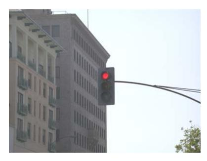
**DESCRIPTION:** This project provides for the replacement of 8-inch and 12-inch incandescent traffic signal indicators with 12-inch light-emitting diode (LED) indicators along various routes.
