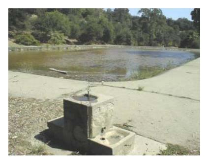
**DESCRIPTION:** This project will repair the casting pond. The pond is for the practice of fly casting and other appropriate uses by local residents, as well as organized groups. Repairs will include the construction of a new drain, installation of reinforced membrane, removal of asphalt decking, construction of pond curbing and the construction of a maintenance ramp into the pond.
