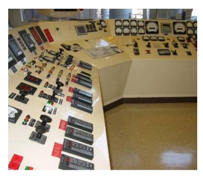
**DESCRIPTION:** This ongoing project will replace obsolete pneumatic analog instruments and controls at the Broadway and Glenarm Power Plants with solid state and digital equipment, and provide new and upgraded metering, monitoring, control, and communication equipment. Discrete instruments and controls will be replaced on an as-needed basis.
