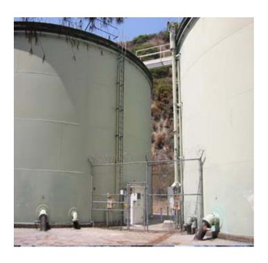
**DESCRIPTION:** This project will provide for major repairs and upgrades to the City's 15 existing water tanks and reservoirs. Most of the tanks and reservoirs are over 60 years old. Examples of the repairs and upgrades may include replacement of reservoir roofing, lining the reservoir floor with hypaton liners, and changing old outlet and inlet valves.
