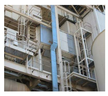
**DESCRIPTION:** This project provides for emission reduction in oxides of nitrogen from Broadway Unit B-3 through periodic replacement of the spent catalyst in the Selective Catalytic Reduction (SCR) system.
