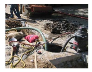
**DESCRIPTION:** This project provides for the closed-circuit television inspection and appropriate rehabilitation of the sewer in Laguna Road between Hermosa Road and Arroyo Boulevard.
