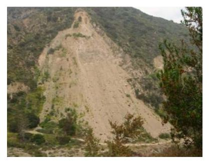
**DESCRIPTION:** This project provides for the repair of a portion (about 0.5 mile) of Mount Wilson Toll Road within the City of Pasadena boundary, and debris cleanup from the large landslide in Eaton Canyon. Work will be completed by Los Angeles County Fire Department, the main user of the road.
