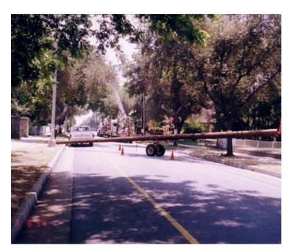
**DESCRIPTION:** This project provides for the testing of wood utility poles for structural soundness and wood decay with resulting replacement or reinforcement as required. It also provides for the replacement of overhead circuit conductors as required.
