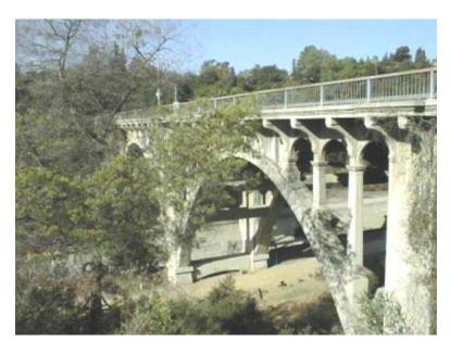
**DESCRIPTION:** The project provides for the rehabilitation of the La Loma Road Bridge that spans the Arroyo Seco at La Loma Avenue. The rehabilitation of the bridge includes seismic retrofitting, repair of deteriorated and damaged surfaces, and replication of the historical lighting and bridge rail features.
