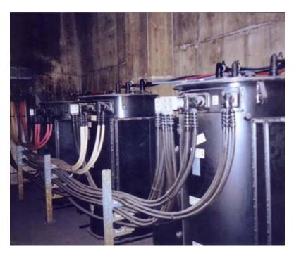
**DESCRIPTION:** This project provides for the installation of high and low voltage cables, transformers, switches, and other equipment in a vault or enclosure provided by the customers on their own property.
