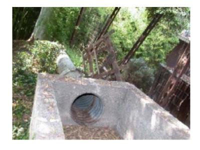
**DESCRIPTION:** This project provides for the inspection and systematic lining or replacement of portions of corrugated metal pipe (CMP) storm drains throughout the City. The City has 6,456 lineal feet of CMP storm drains that were installed from 1925 to 1953. Several of these drains are rusted and are in immediate need of repair.
