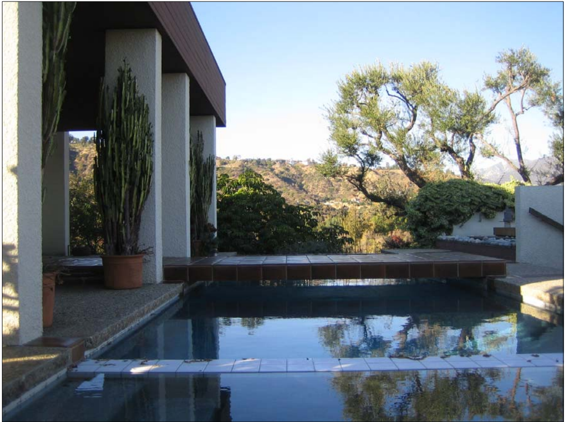
Pool & walkway from south
