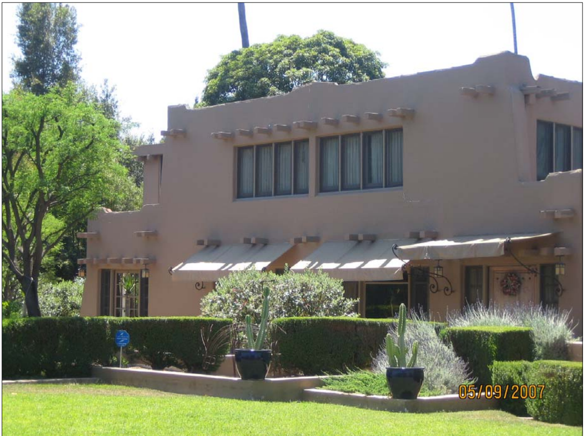
Southern portion of east elevation
