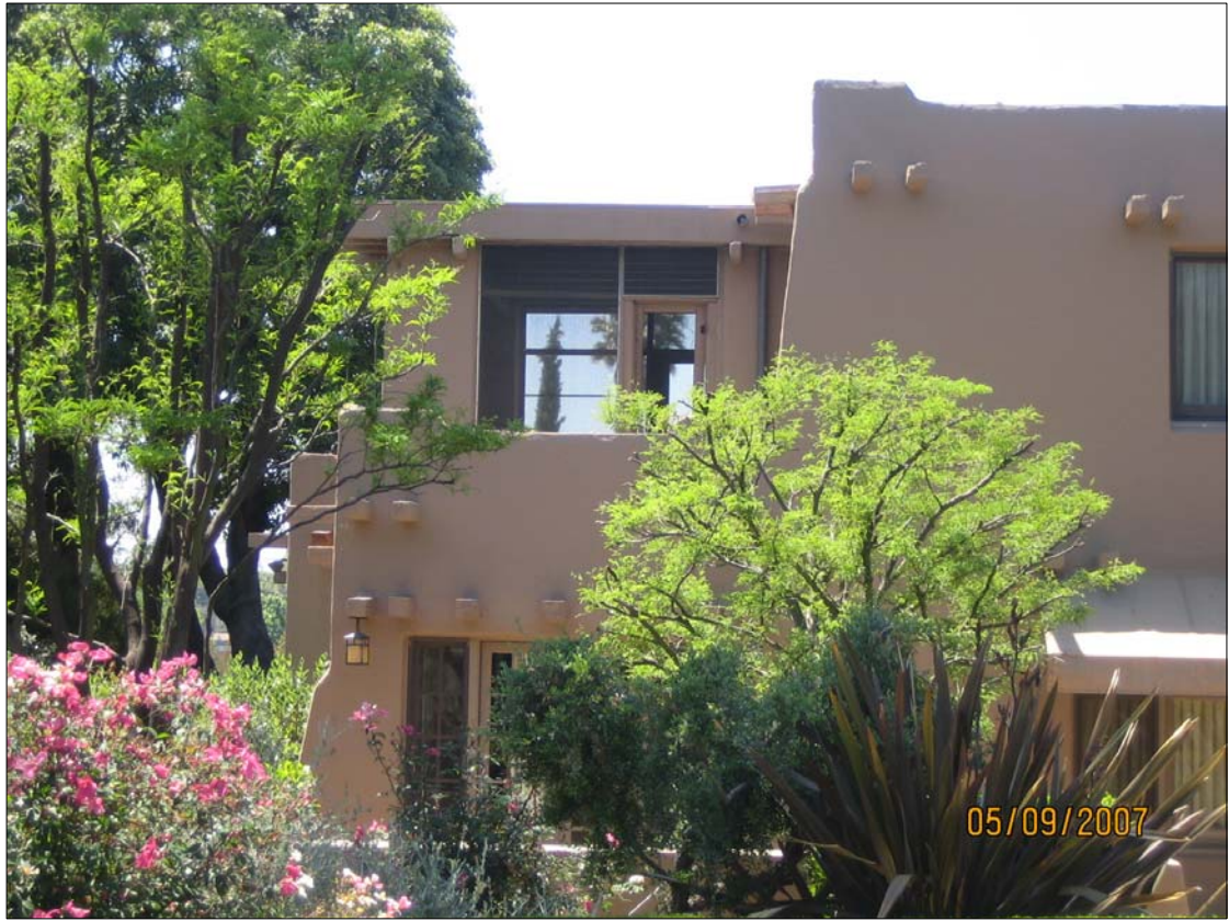
Possible addition – southeast corner
