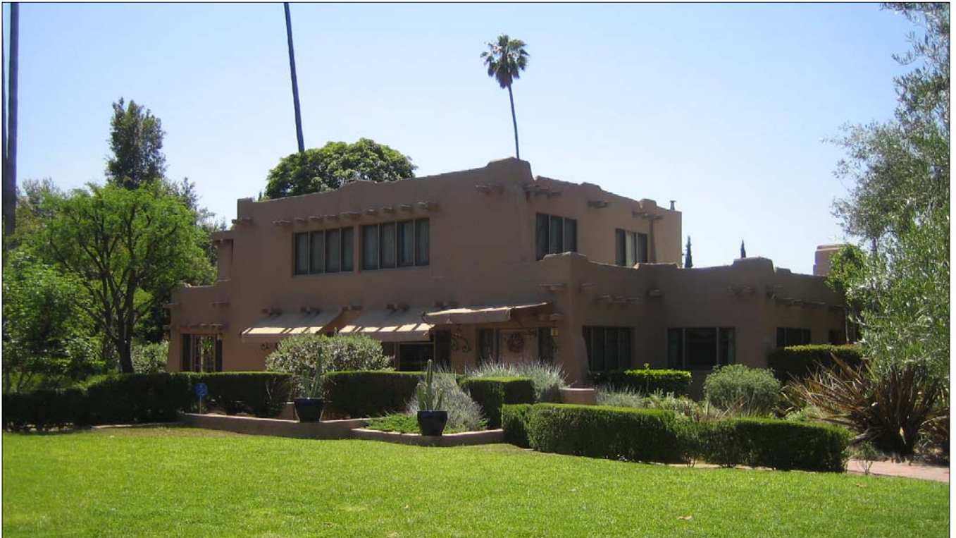
East (S. Oakland Avenue) elevation
