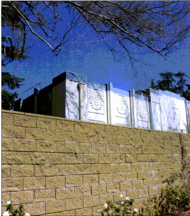
Visible portion of west elevation
