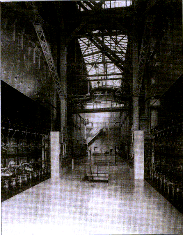
Boiler Room hallway (east end – now empty)
