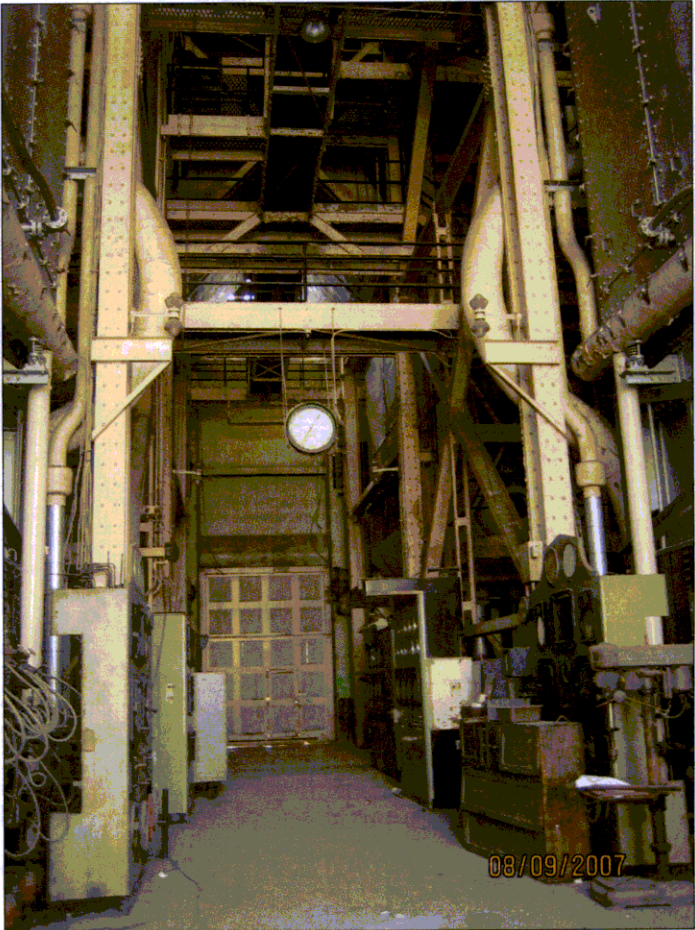
Boiler Room hallway (west end - current)
