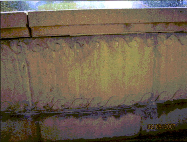
Fountain perimeter wall detail
