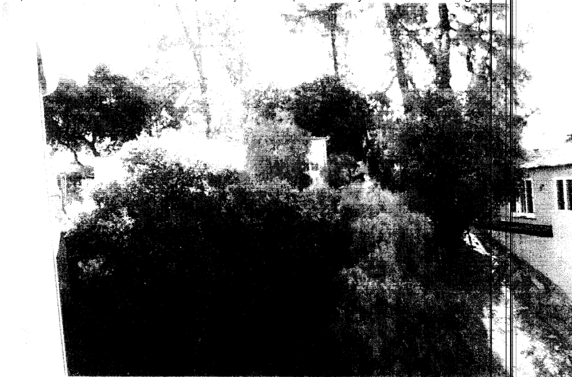
Figure 15- House, from upper left of Figure 14, at top of slope with dry, flammable. Different view.
