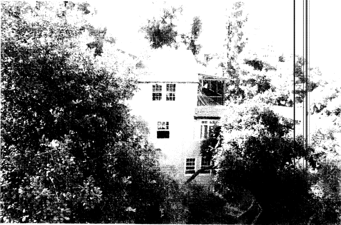
Figure 11- Overview showing significant flammable vegetation within project area.
