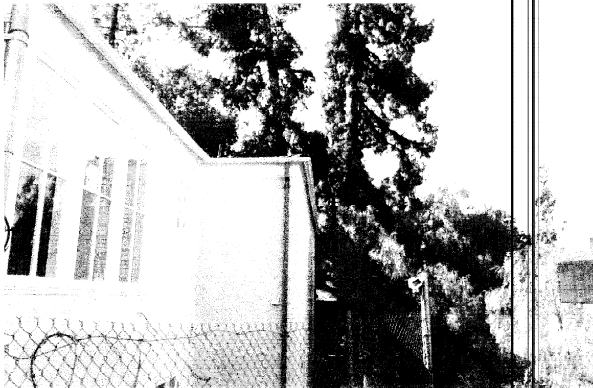
Figure 6- Structure with unpermitted wood roof immediately adjacent flammable brush on slope (see also Figure 7)
