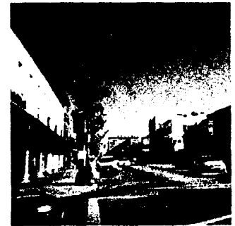
Downtown Precedent: a consistent building frontage defines the space of the street
