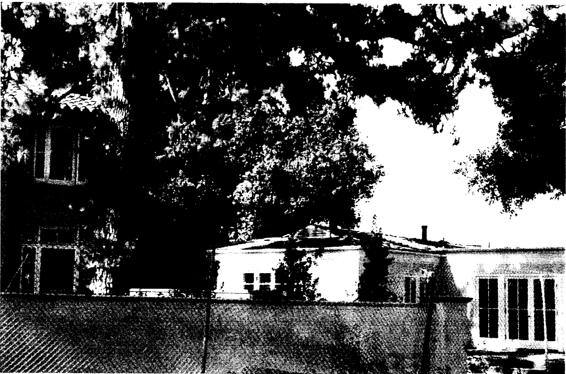
Figure 4- Flammable vegetation over and amongst unpermitted wooden roofs and permitted tile roof.
