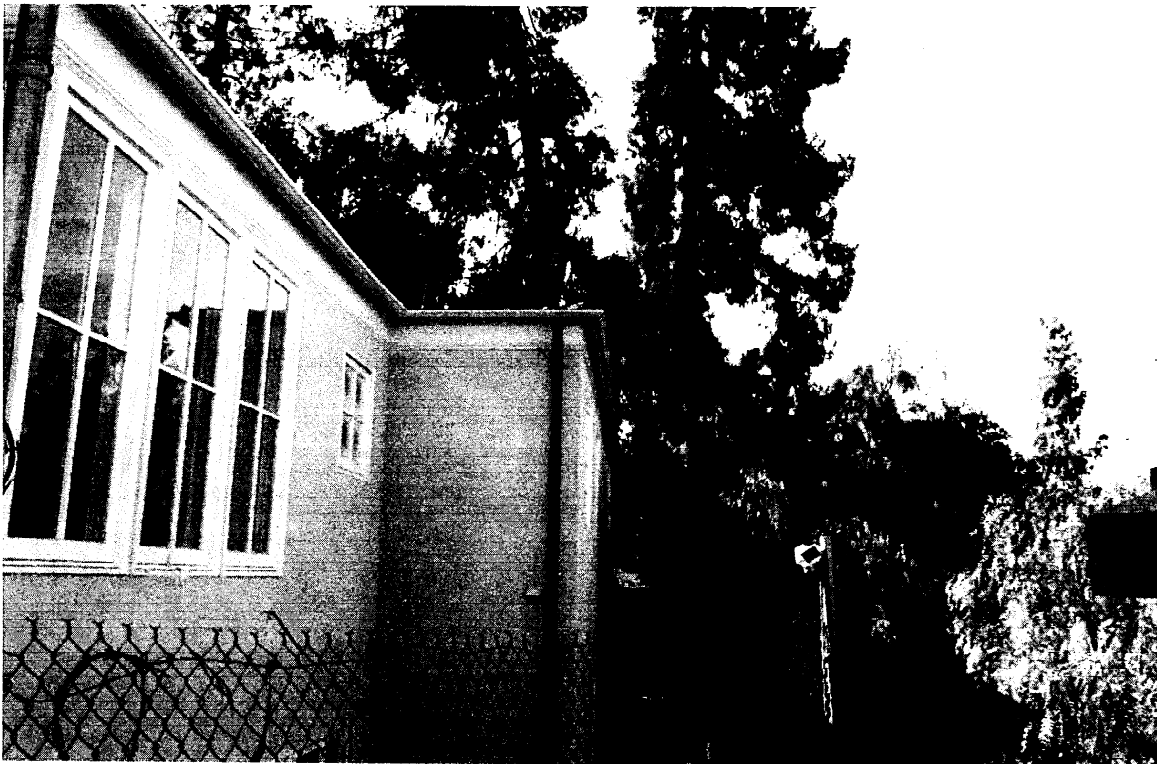
Figure 6- Structure with unpermitted wood roof immediately adjacent flammable brush on slope (see also Figure 7)
