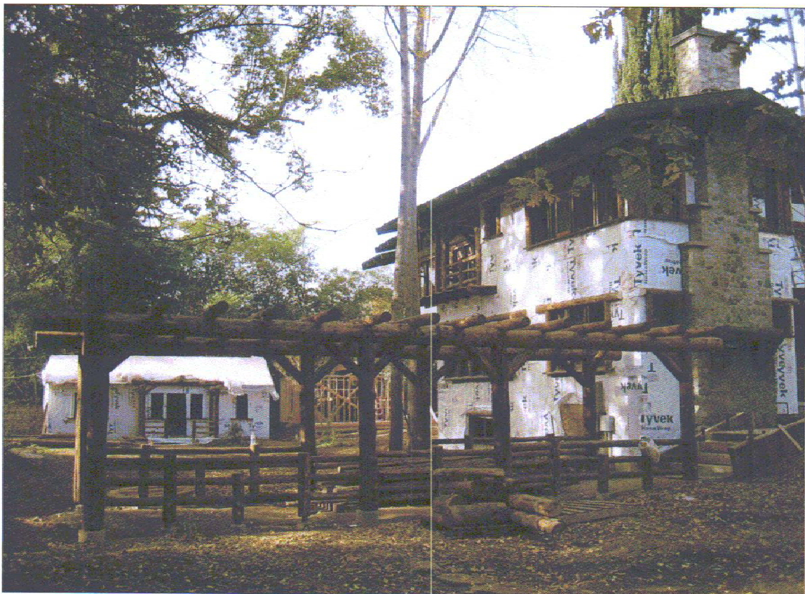
South side of street elevation under restoration
