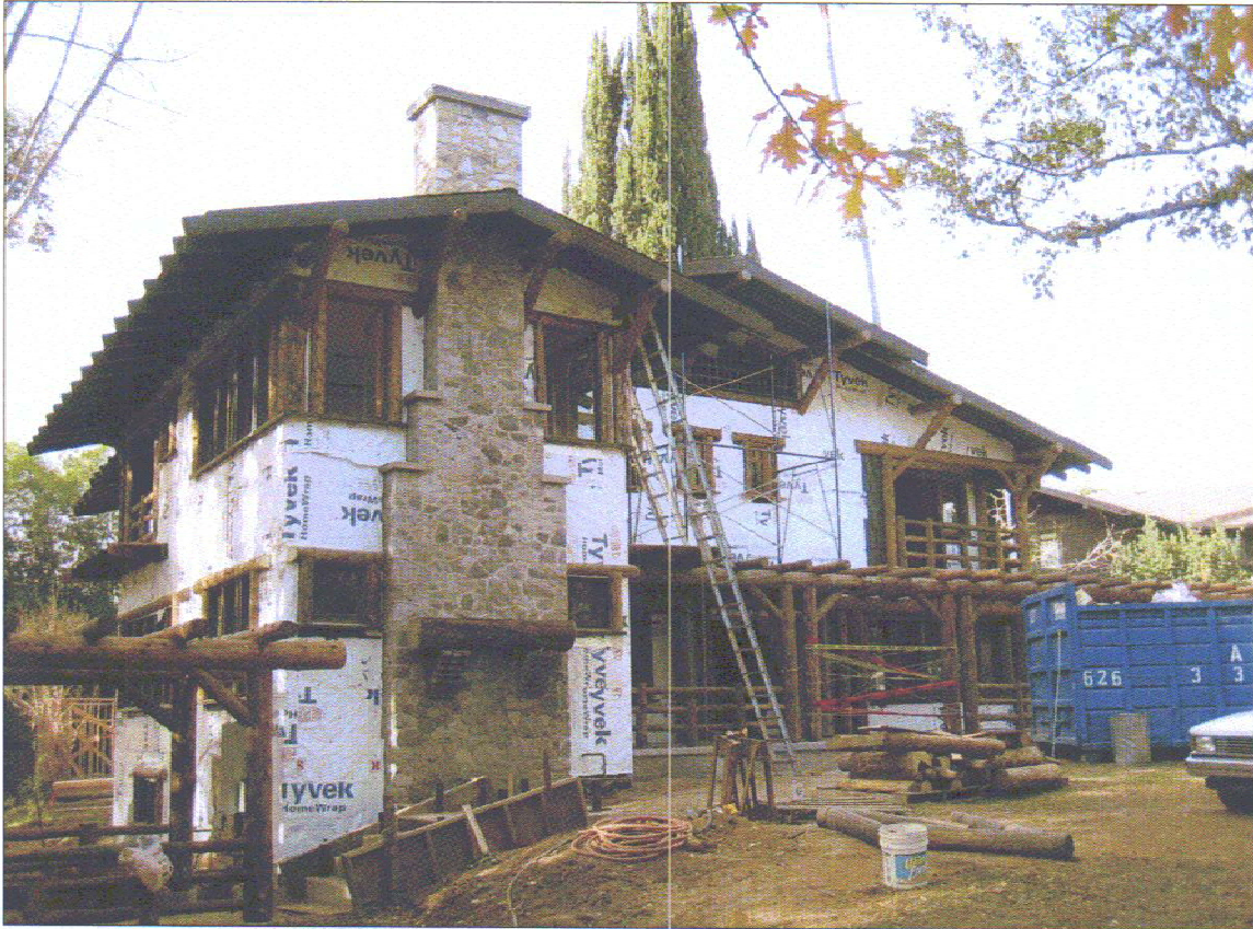
North side of street elevation under restoration
