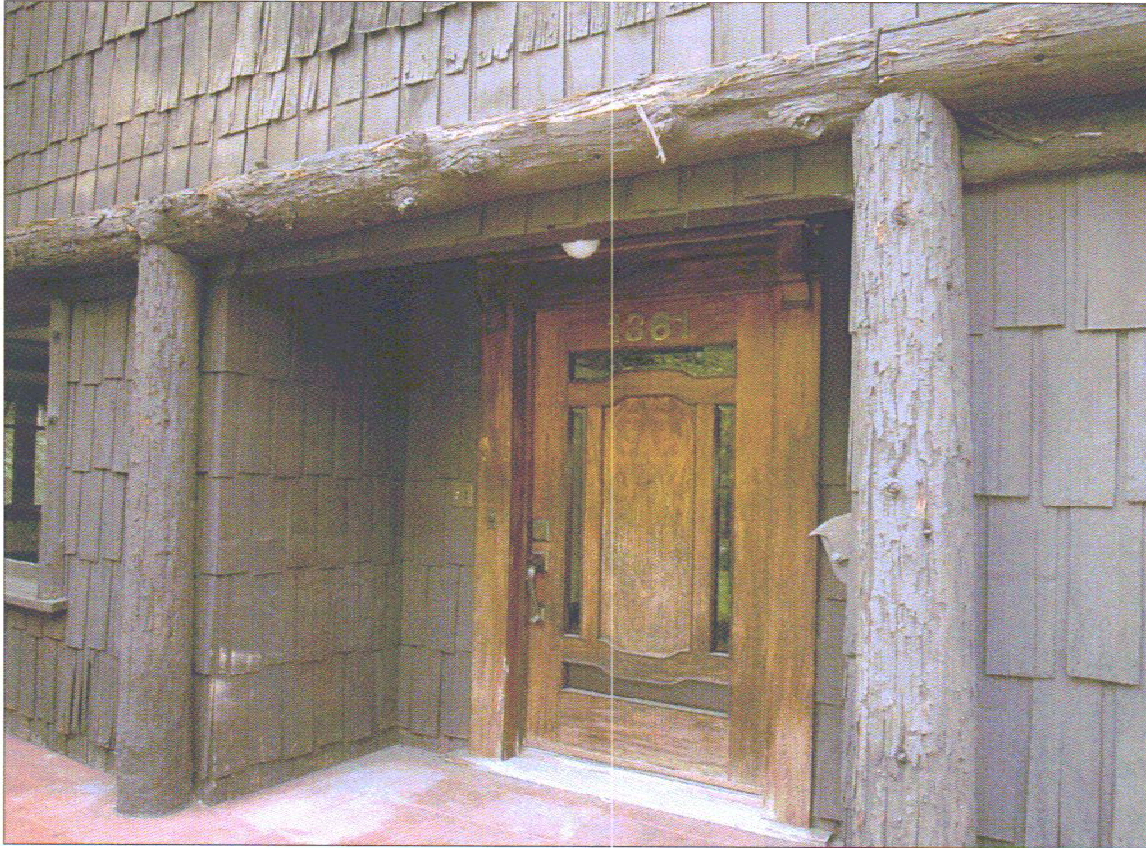
Front door/remaining logs prior to restoration
