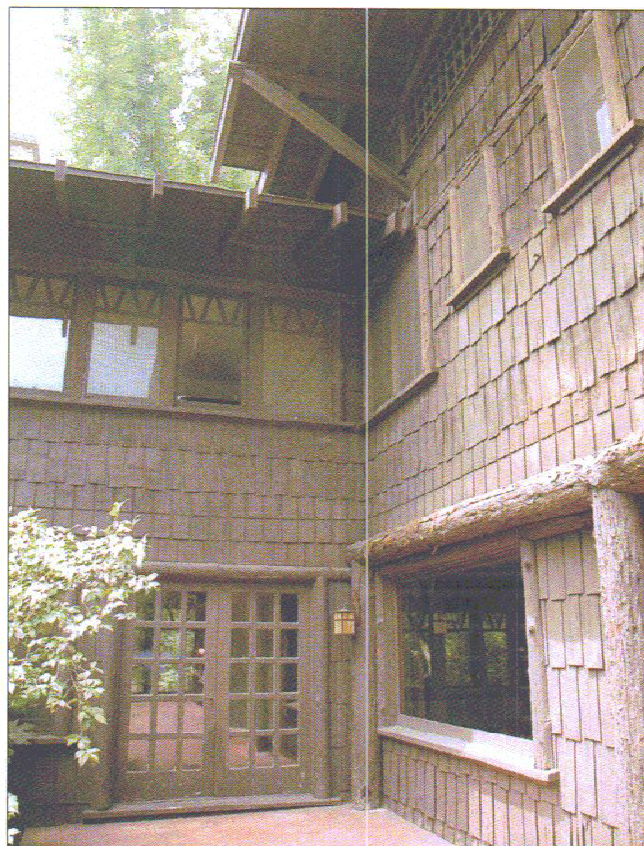
Front porch area prior to restoration
