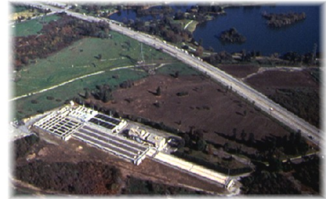
Whittier Narrows Water Reclamation Plant. Image source: Sanitation Districts of Los Angeles County
