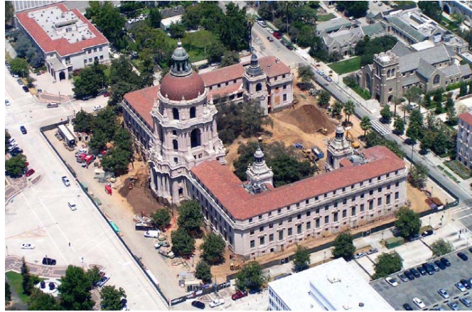
An aerial view of City Hall shows the temporary one-way sections of Garfield Ave. and Euclid Ave.
