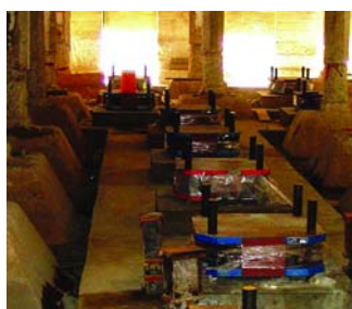
240 base isolators have been installed between the foundation and basement
