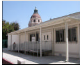
Modular Complex 280 Ramona St. (next to Permit Center)
