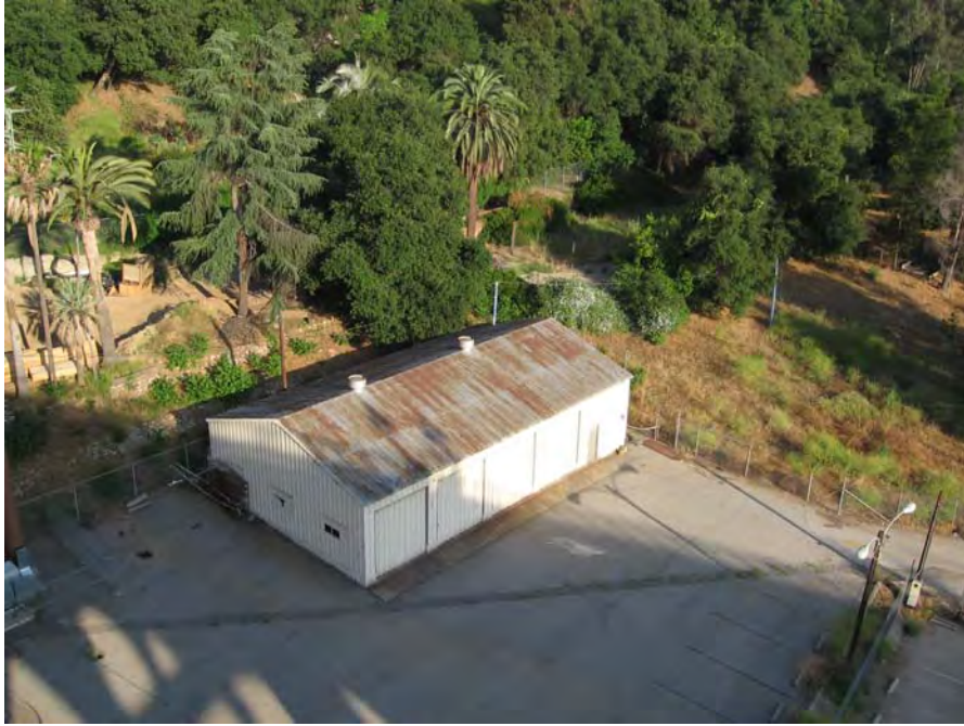
View of Garage from Colorado Bridge
