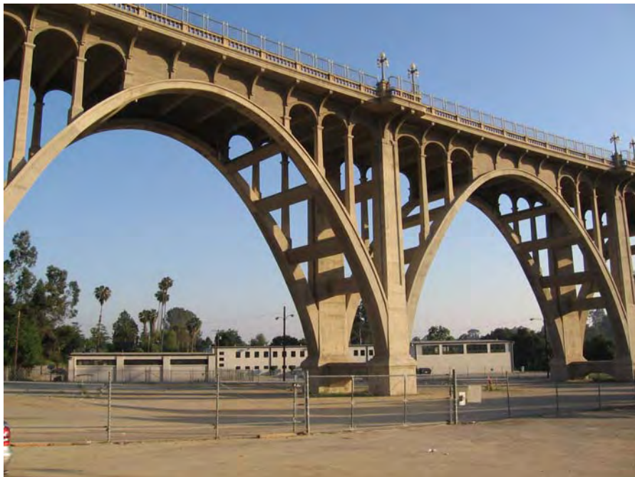
View from Underneath the Colorado Bridge
