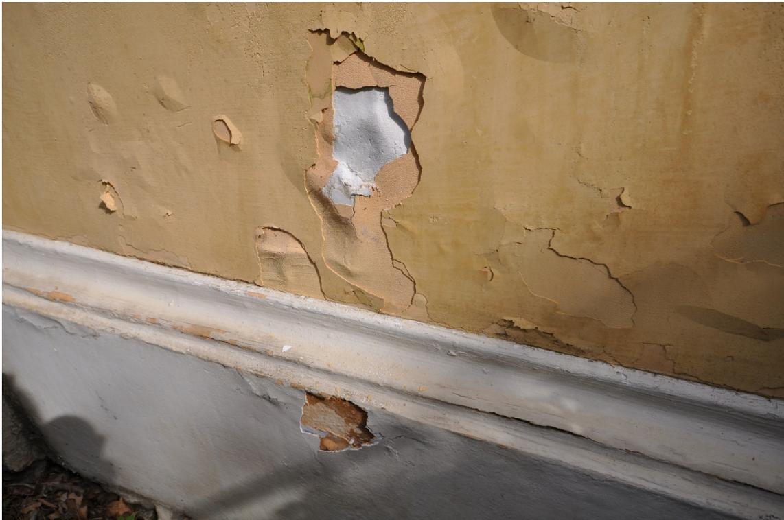
Photo 14: Detail of water damage on concrete and plaster retaining wall at south elevation terrace. View looking northwest. April 2020. GPA.
