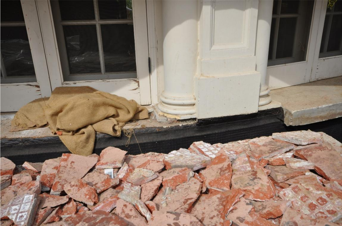
Photo 18: Detail of tile removed on east terrace for waterproofing of foundation. April 2020. GPA.
