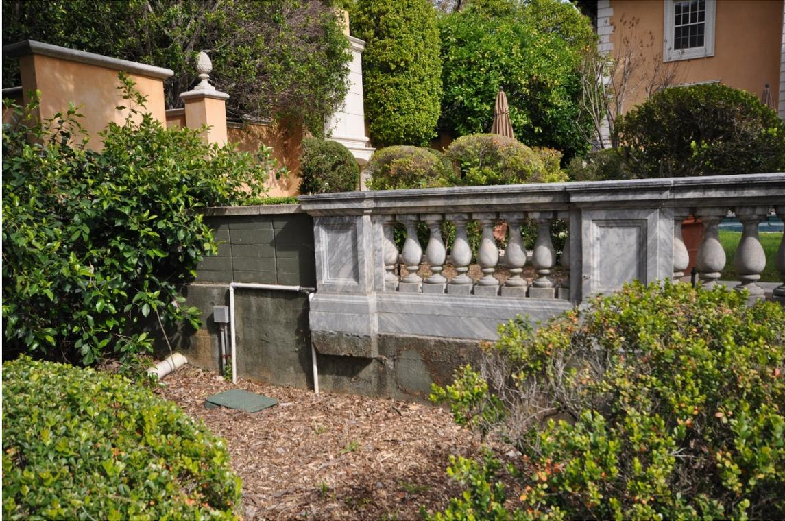
Photo 13: Detail of marble balustrade and concrete wall (non-original) in south yard. View looking northwest. April 2020. GPA.
