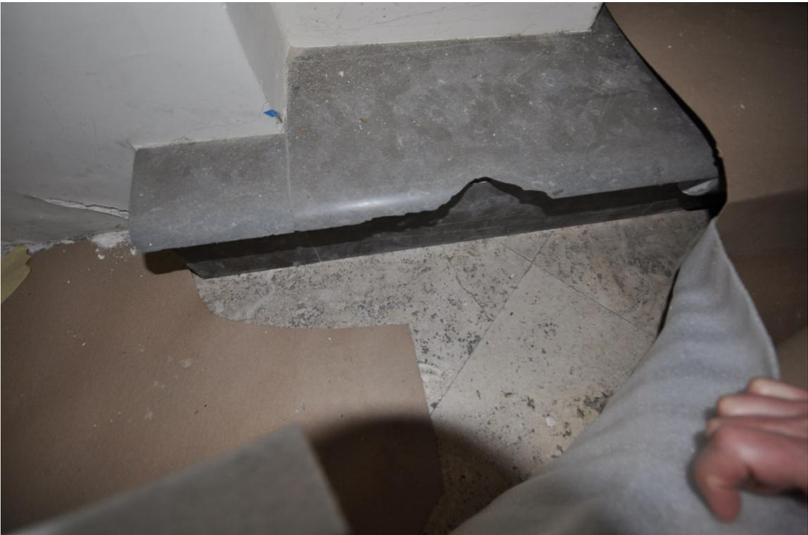
Photo 34: Sunroom. Detail of chipped stone step showing travertine floor. April 2020. GPA.
