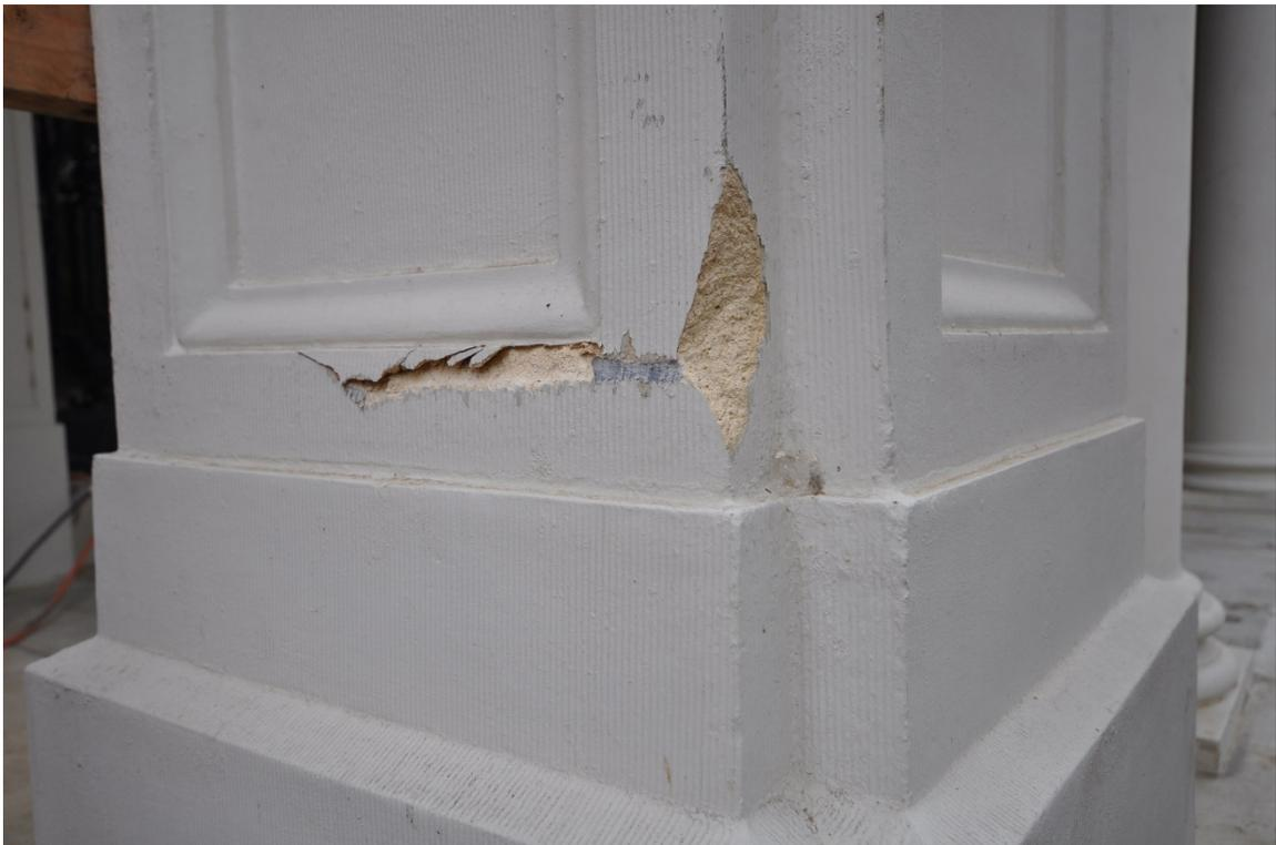
Photo 8: Detail of damaged concrete. Main entrance column. April 2020. GPA.
