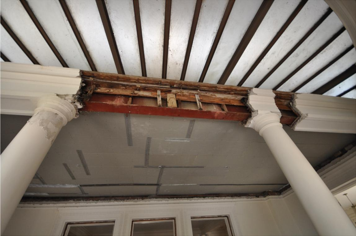
Photo 33: Sunroom. Detail of exposed structural beam at copper skylight. View looking west. April 2020. GPA.
