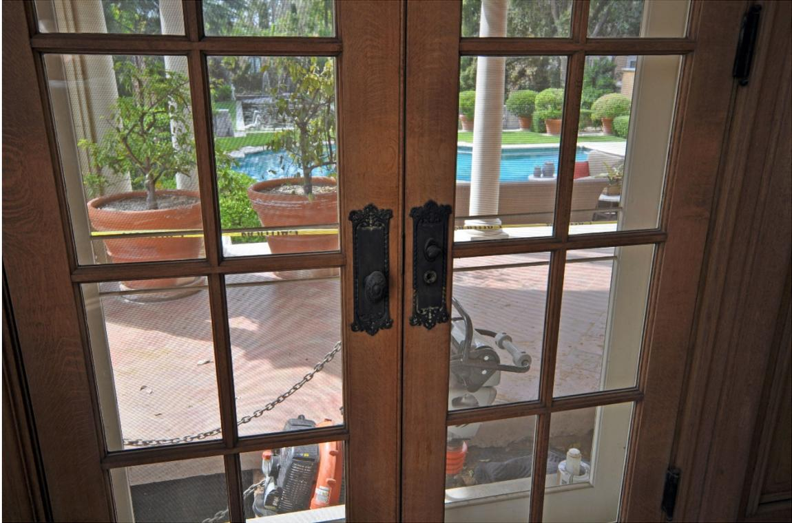
Photo 31: Living room. Detail of French doors showing missing hardware. View looking south April 2020. GPA.
