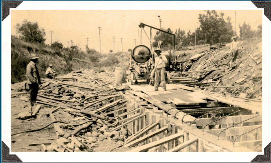
Storm Drain Under Construction, 1916
