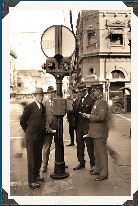
Installation of New Traffic Signal, 1928
