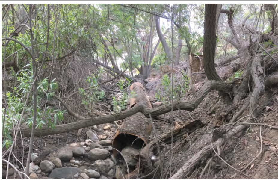
Photo Location 6, facing upstream. May 25, 2018. View of metal drain pipes that are debris in Berkshire Creek.
