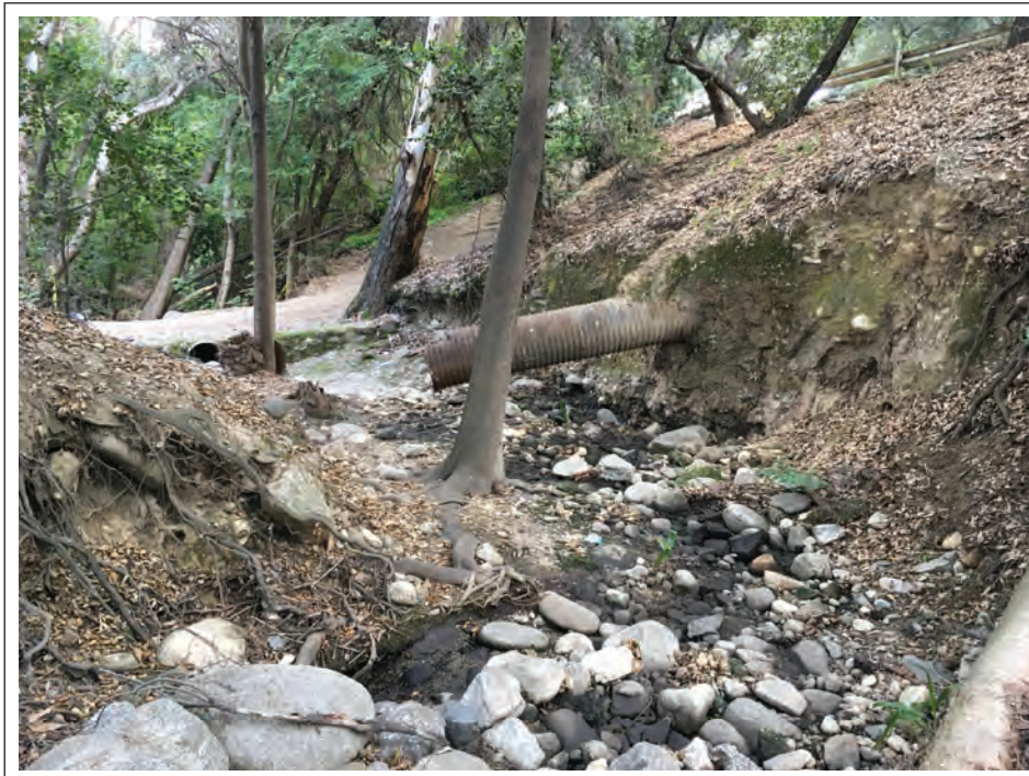
Photo Location 3, facing downstream. May 25, 2018. View of eroded right bank of Berkshire Creek and exposed metal drain pipe.
