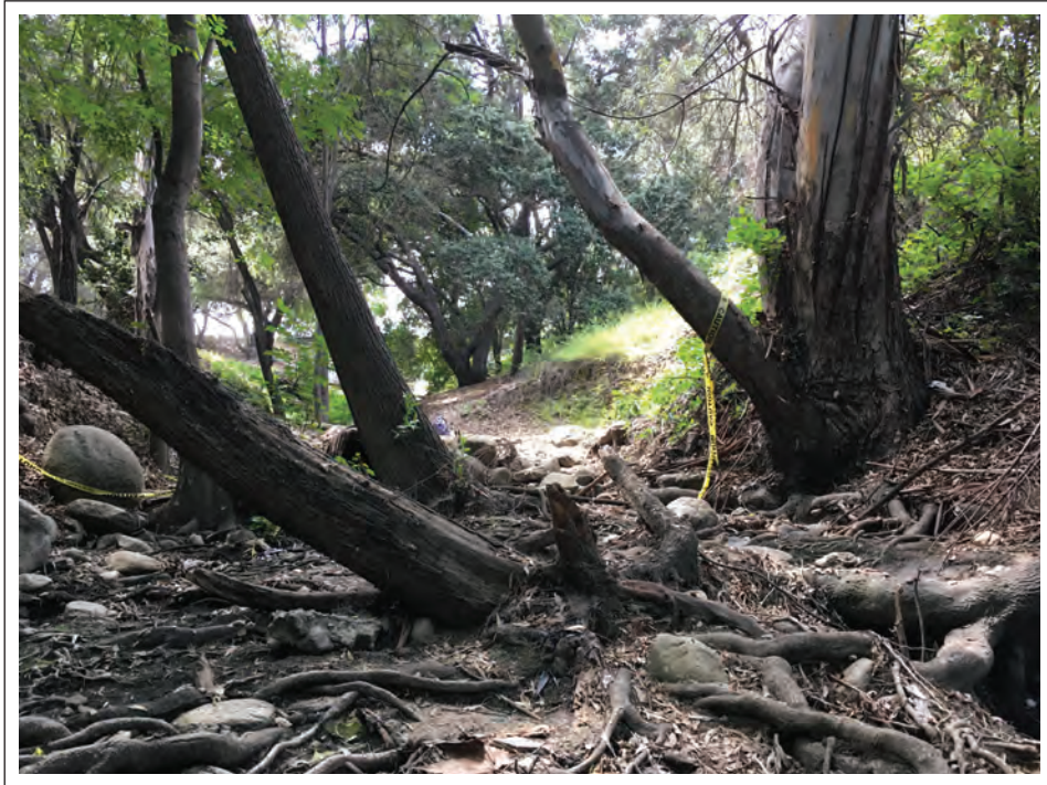
Photo Location 5, facing upstream. May 25, 2018. View of eroded streambed in lower portion of Berkshire Creek.
