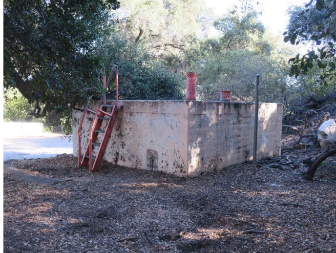
Concrete utility structure (post-1970) near equestrian picnic area, view to southeast. ARG, 2018.
