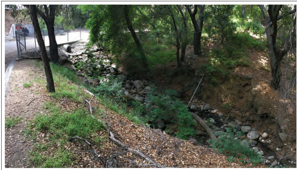
Photo Location 1. May 25, 2018. Overview of upper Berkshire Creek.
