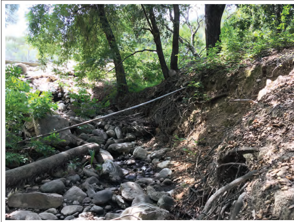
Photo Location 3, facing upstream. May 25, 2018. View of heavily eroded left bank of upper Berkshire Creek.
