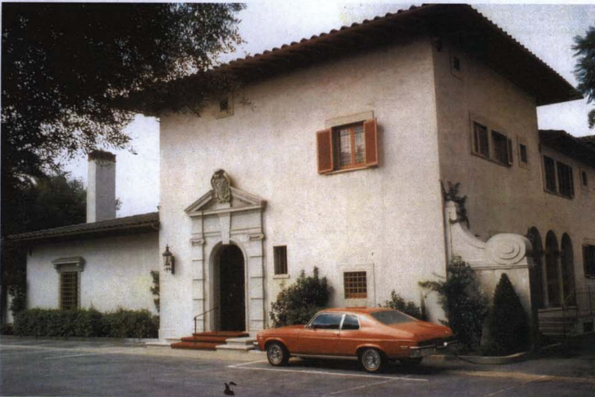
PHOTOGRAPH SHOWING THE ORIGINAL BUILDING CONDITION WITH WOOD SHUTTERS AND A DECORATIVE CHIMNEY HOOD
