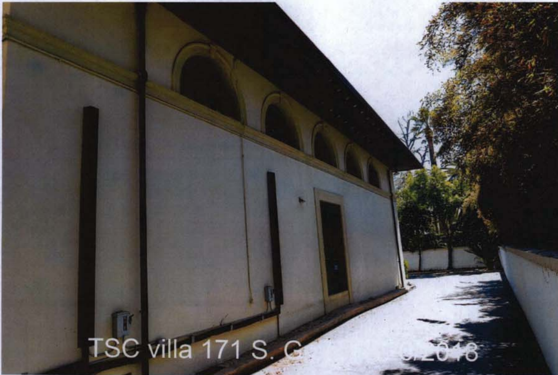
VIEW LOOKING SOUTHEAST AT THE WESTERLY FACADE
