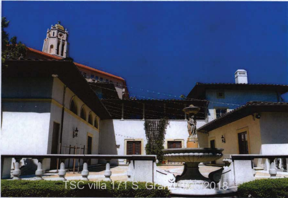
VIEW LOOKING NORTH AT THE PATIO. LOGGIA IS VISIBLE ON THE SECOND STORY
