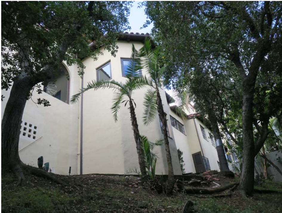
North elevation and projecting bay, view southwest.
