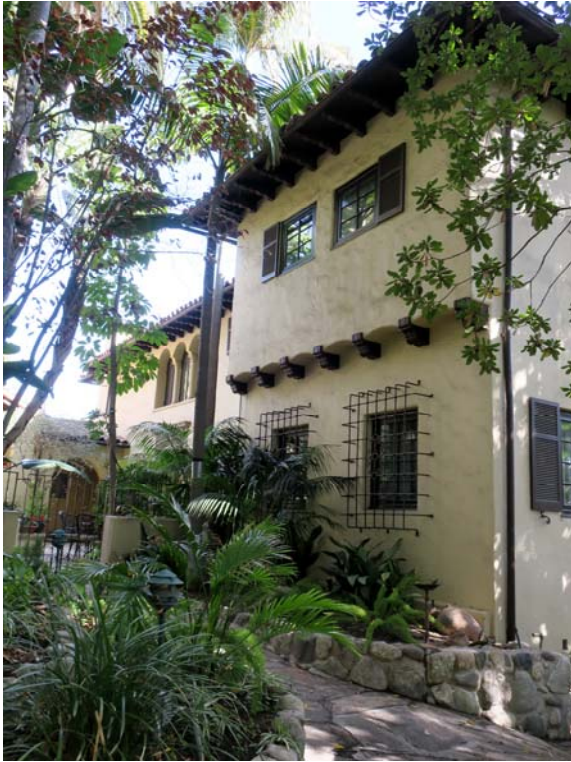
Primary (west) elevation, view northeast.
