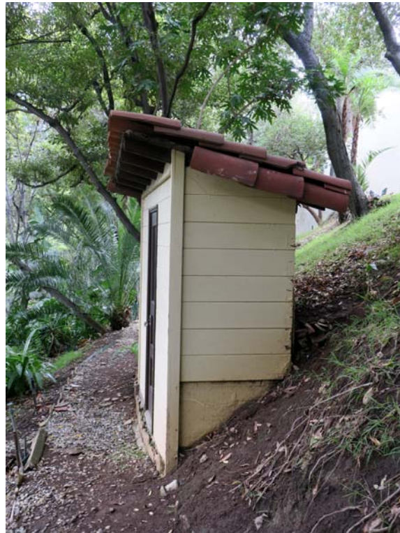
Storage shed (north of house), view southwest.
