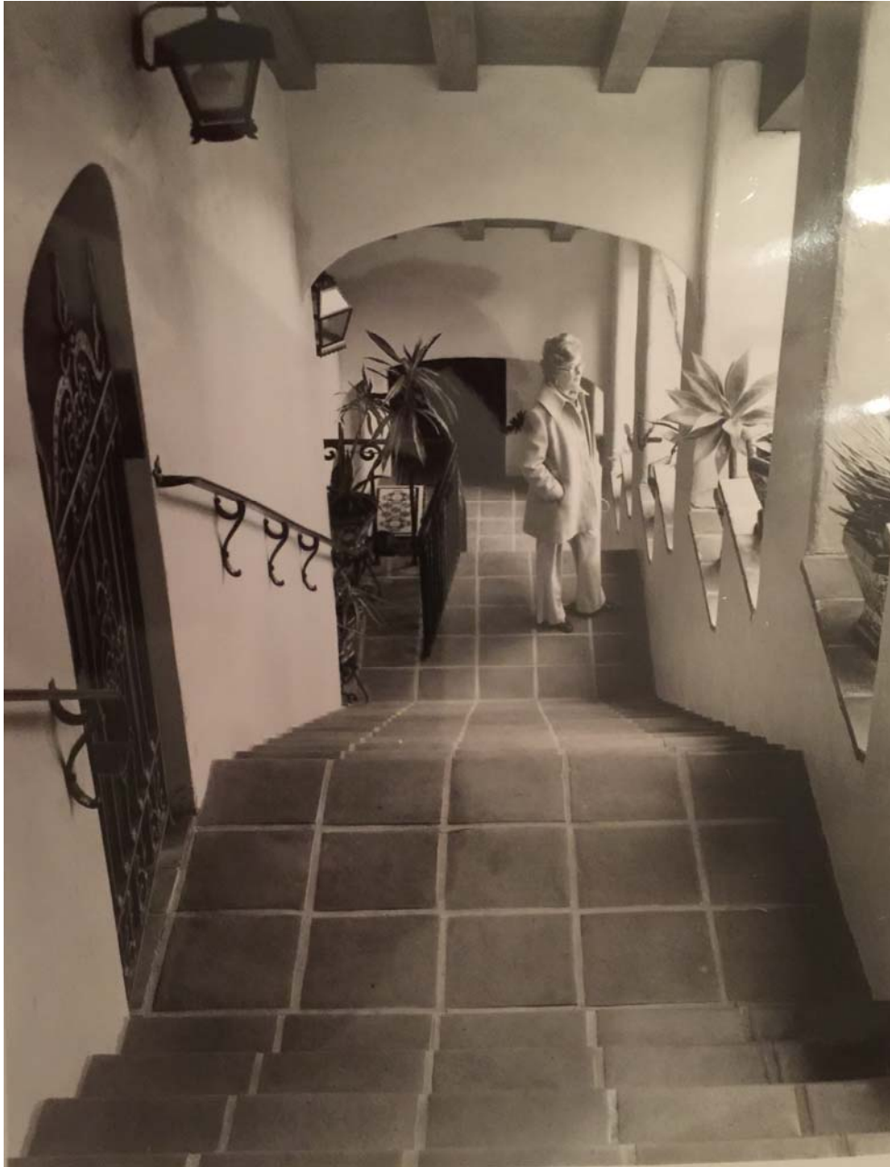
Entrance stairwell with quarry tile, n.d. (courtesy Mihaela Varga).
