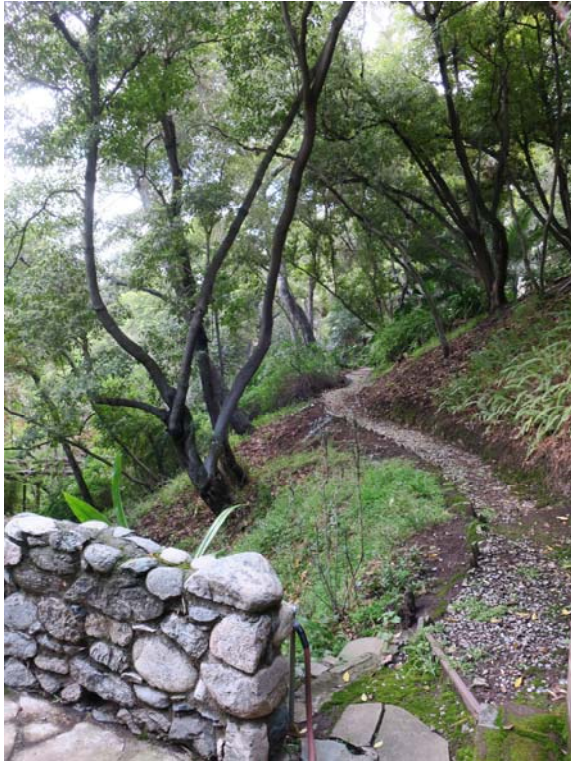
Arroyo stone retaining wall and dense vegetation (north of house), view east.
