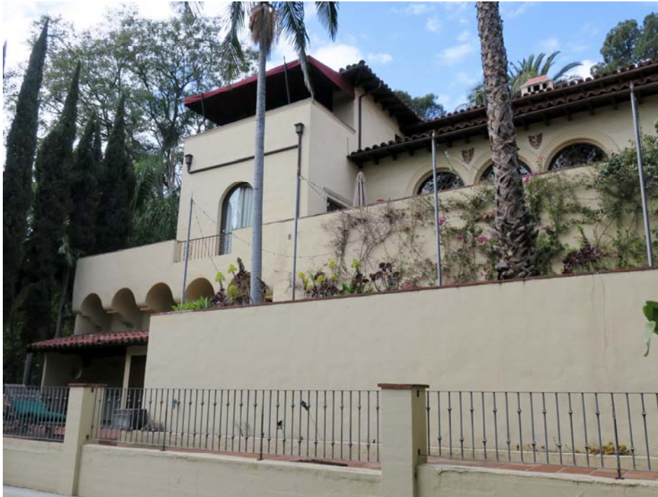
Rear (east) elevation as viewed from pool terrace, view southwest.
