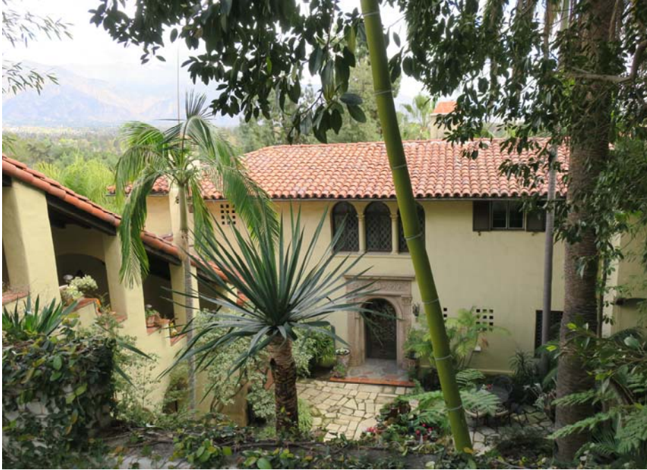
Primary (west) elevation as viewed from street level, view northeast.
