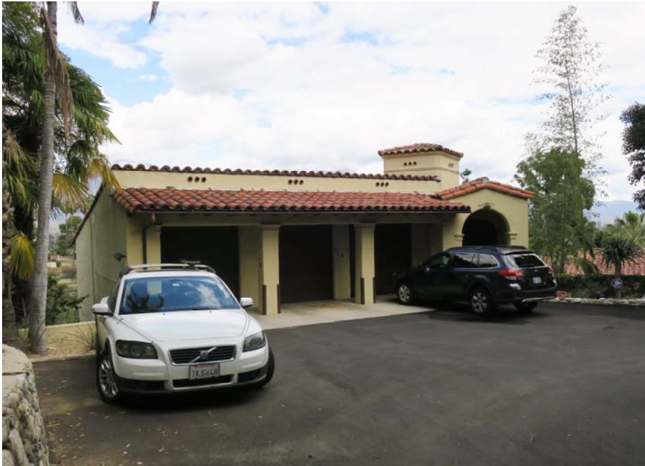
Garage at street level, view northeast.
