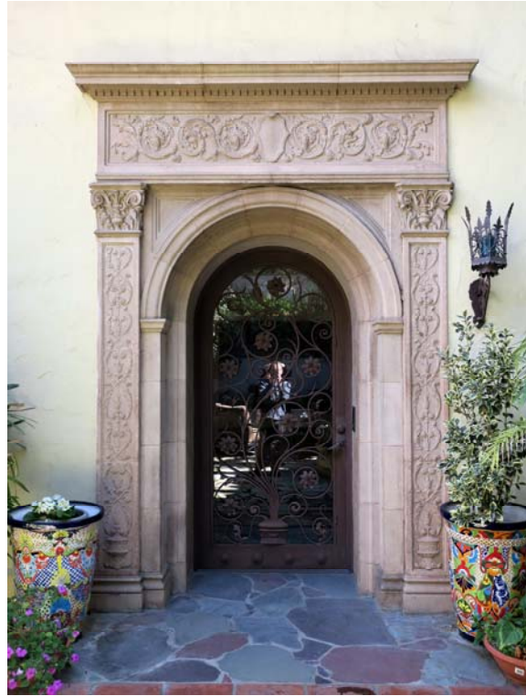
Articulated entrance and surround on primary elevation, view east.
