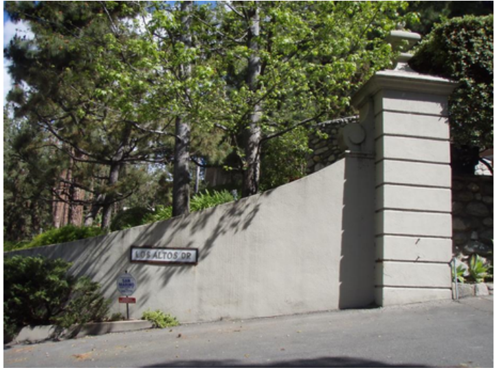
Description: Entry gate & sign Photo Date: 04/08/2011
