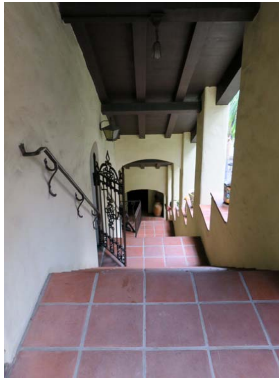
Exterior stairwell with quarry tile, leading from the street to the house, view east.
