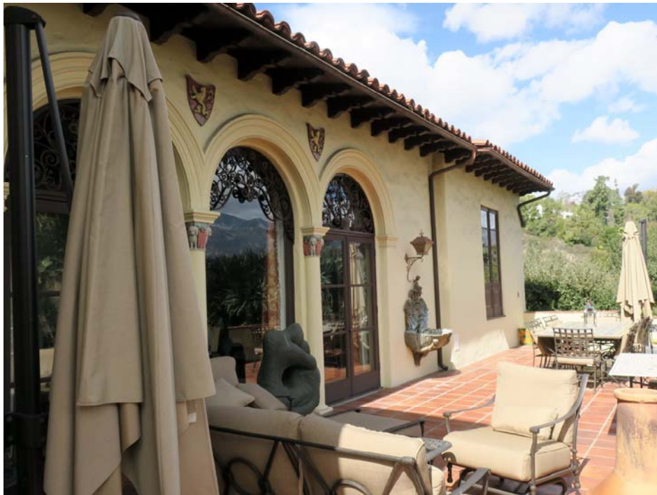
Rear elevation as viewed from upper terrace, view northwest.
