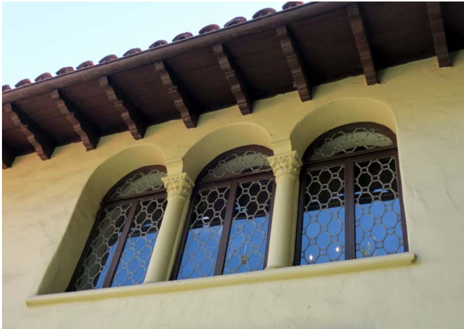
Detail of decorative wood brackets, accent windows, and colonettes on primary elevation.
