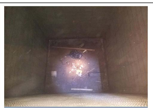
Photograph 3: View of the inside of the anechoic tank. Water or other indications of liquid were not observed.
